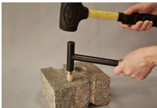
Figure 2. Installing the Vapor Pin™.
