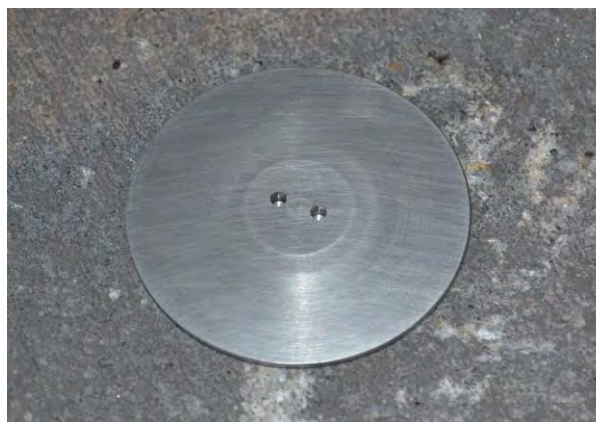
Figure 4. Secure Cover Installed
