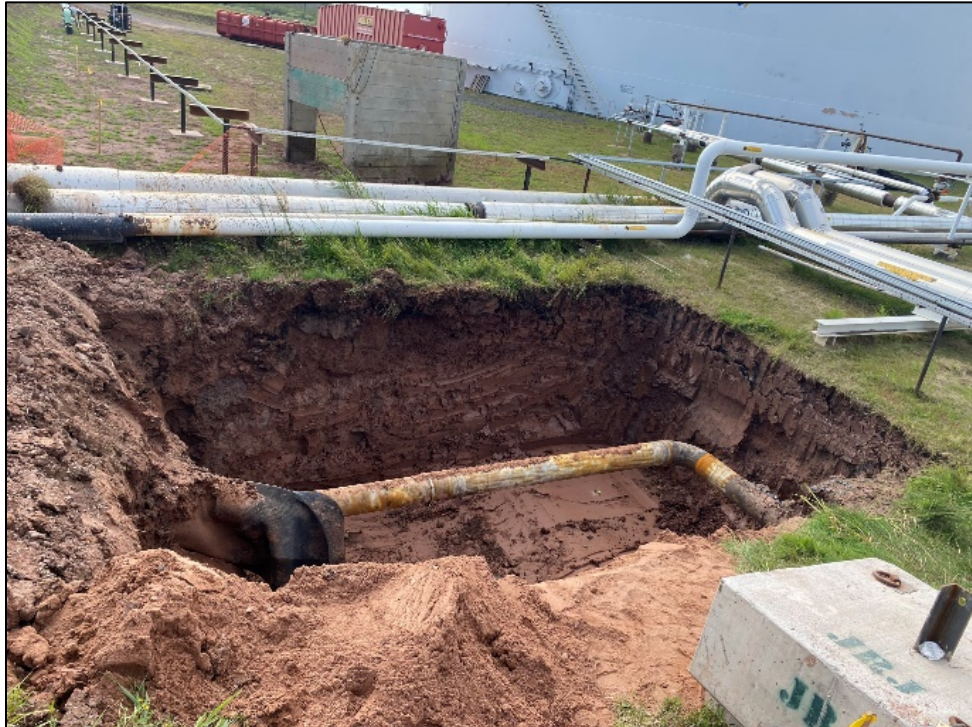
Photo 6 Final excavation extent. Photo taken facing west on August 31, 2021.
