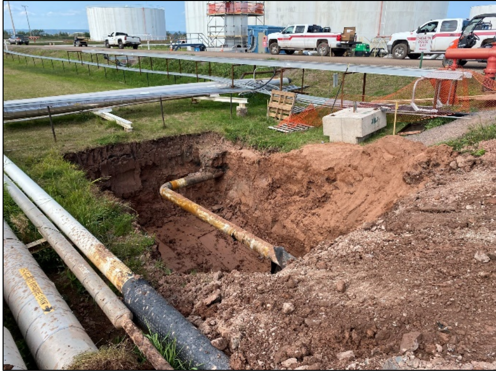
Photo 5 Final excavation extent. Photo taken facing north on August 31, 2021.
