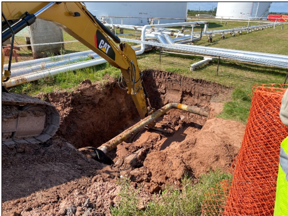
Photo 4 Excavation activities. Photo taken facing northwest on August 31, 2021.
