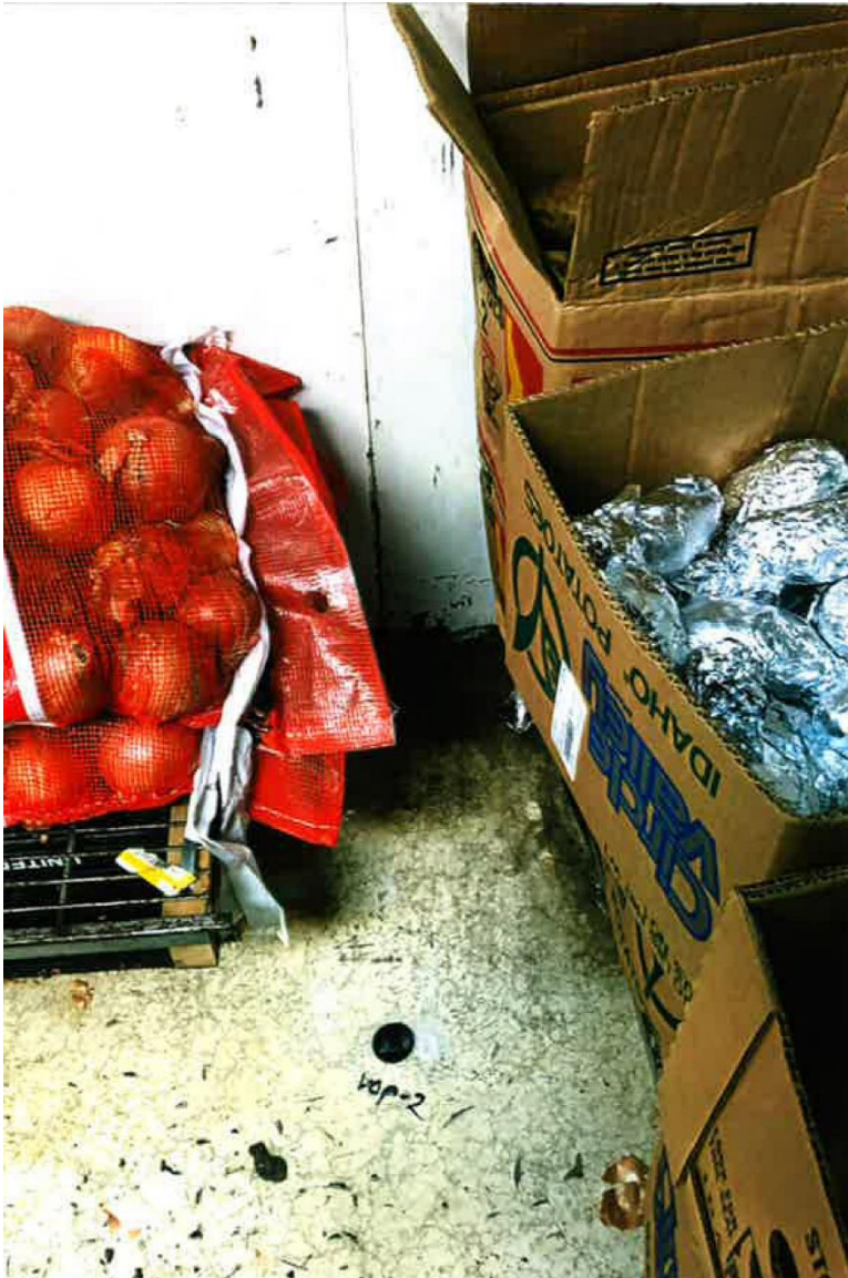
Photo 10: Sub-slab vacuum observation point VOP-2.
