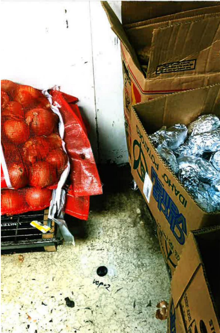
Photo 10: Sub-slab vacuum observation point VOP-2.
