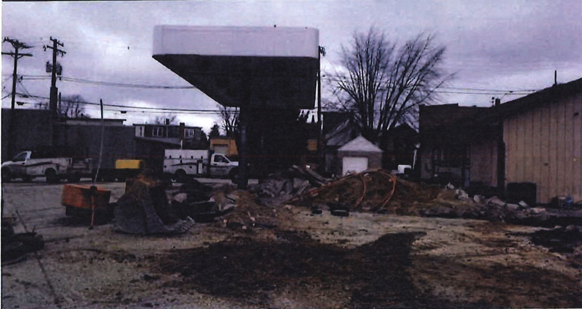
PHOTO 6 – PHOTOGRAPH OF THE CANOPY COVERING THE GASOLINE DISPENSERS
