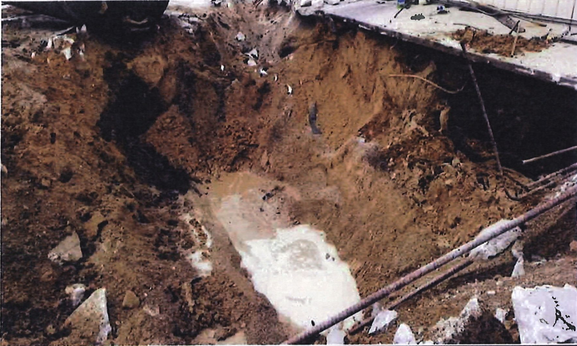
PHOTO 5 – PHOTOGRAPH OF THE EXCAVATION AFTER THE 2 ND 6,000-GALLON TANK WAS REMOVED
