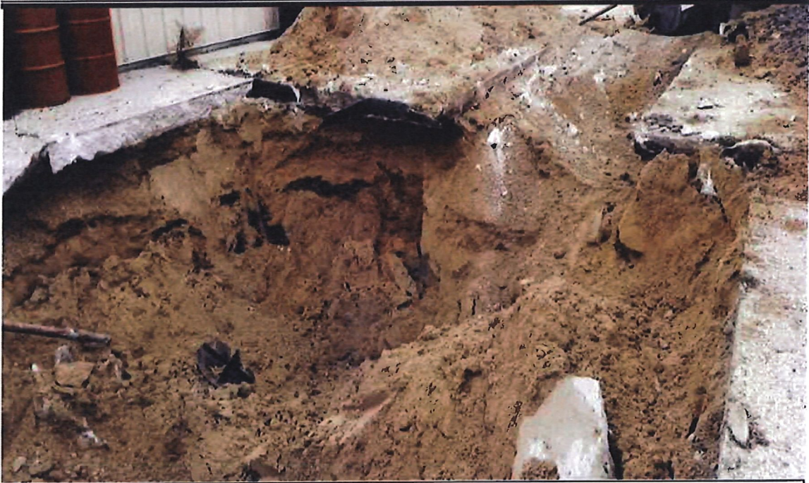
PHOTO 9 – PHOTOGRAPH OF THE NORTHERN TANK EXCAVATION AFTER TANKS WERE REMOVED.
