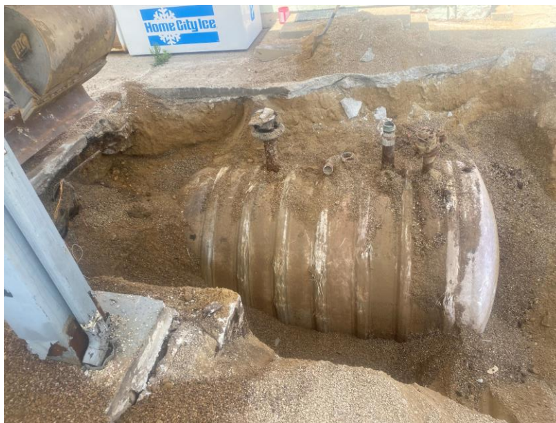
PHOTOGRAPH OF THE 4,000-GALLON UL GASOLINE UST PRIOR TO REMOVAL
