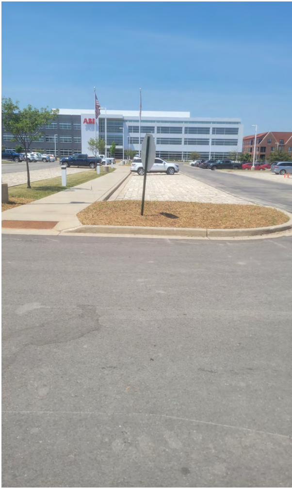
Photo 13: Asphalt paved parking lot within eastern portion of Lot 3 (east of ABB building). Permeable pavers along parking rows of ABB parking lot. Mulched and vegetated topsoil cover within greenspace islands (limited use). View to west; photograph taken on June 1, 2023.
