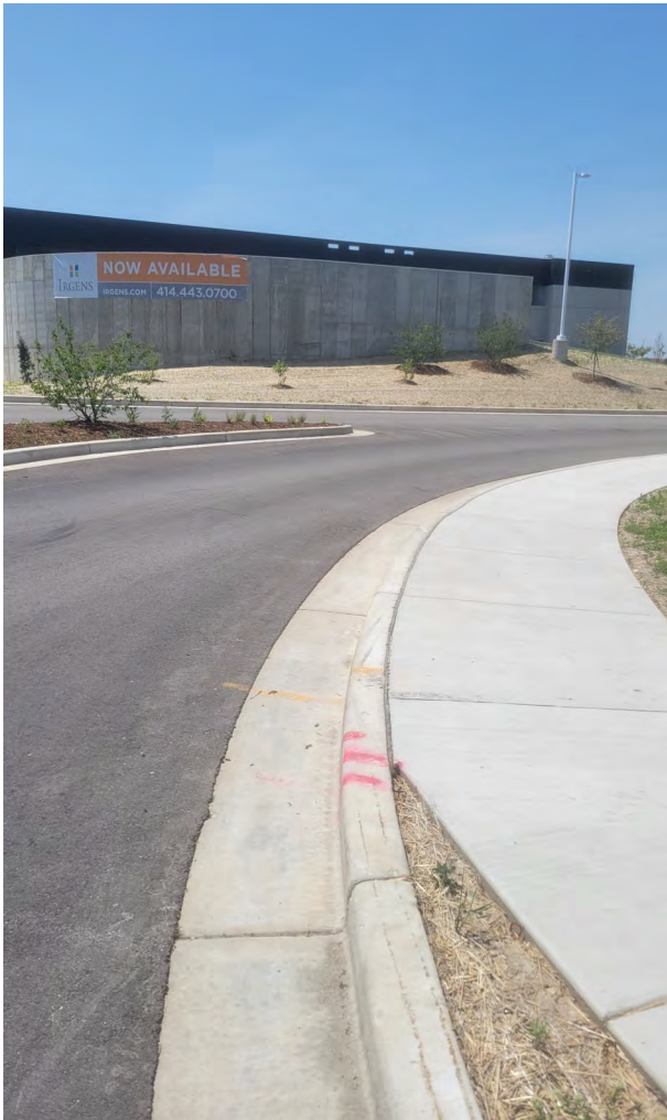
Photo 5: Concrete curb and gutter and sidewalk along the north side of Outlot 3 entrance driveway into the site. Limited greenspace (mulched or grass) within median and along sidewalk. View to southwest; photograph taken on June 1, 2023.
