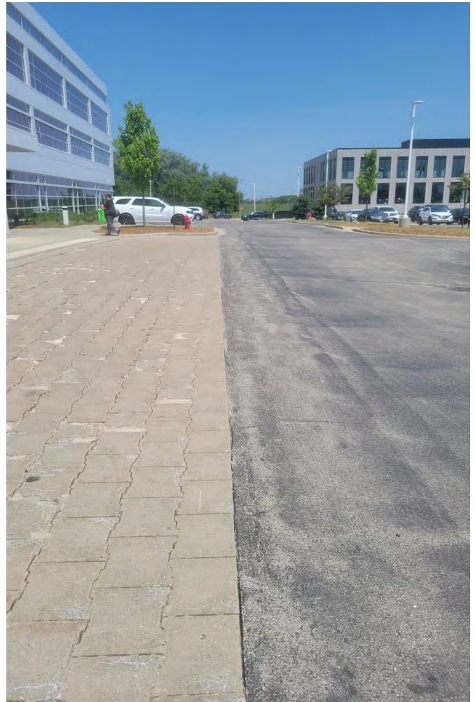
Photo 12: Asphalt paved parking lot within western portion of Lot 3 (east of ABB building). Permeable pavers along parking rows of ABB parking lot. View to north; photograph taken on June 1, 2023.
