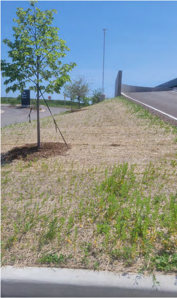
Photo 7: Greenspace along south side of Outlot 3. Cap consists of 6-inches of topsoil with native prairie grass plantings and small trees. Limited use. View to east; photograph taken on June 1, 2023.
