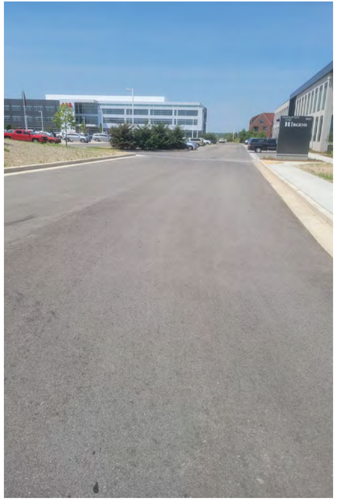
Photo 6: Asphalt paved entrance to Lot 3 and driveway along Building A. Concrete curb and gutter and sidewalk along the south side of Lot 3. View to west; photograph taken on June 1, 2023.
