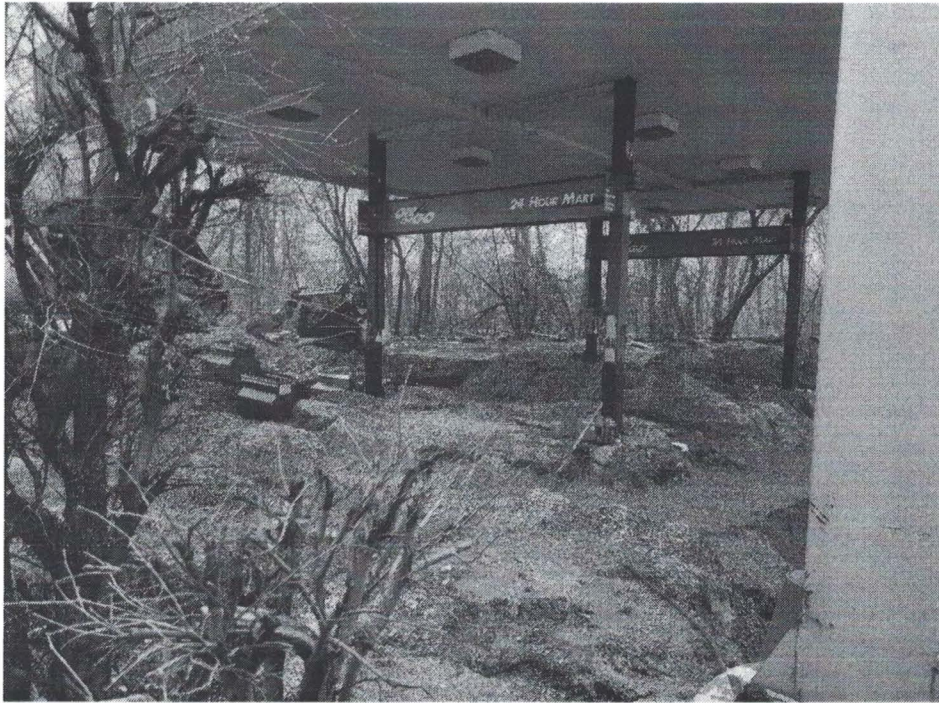
PHOTOGRAPH OF THE FORMER DISPENSER AREA
