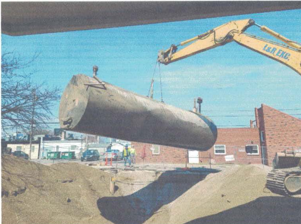
PHOTOGRAPH OF THE SECOND 12,000-GALLON UST JUST AFTER REMOVAL FROM THE EXCAVATION
