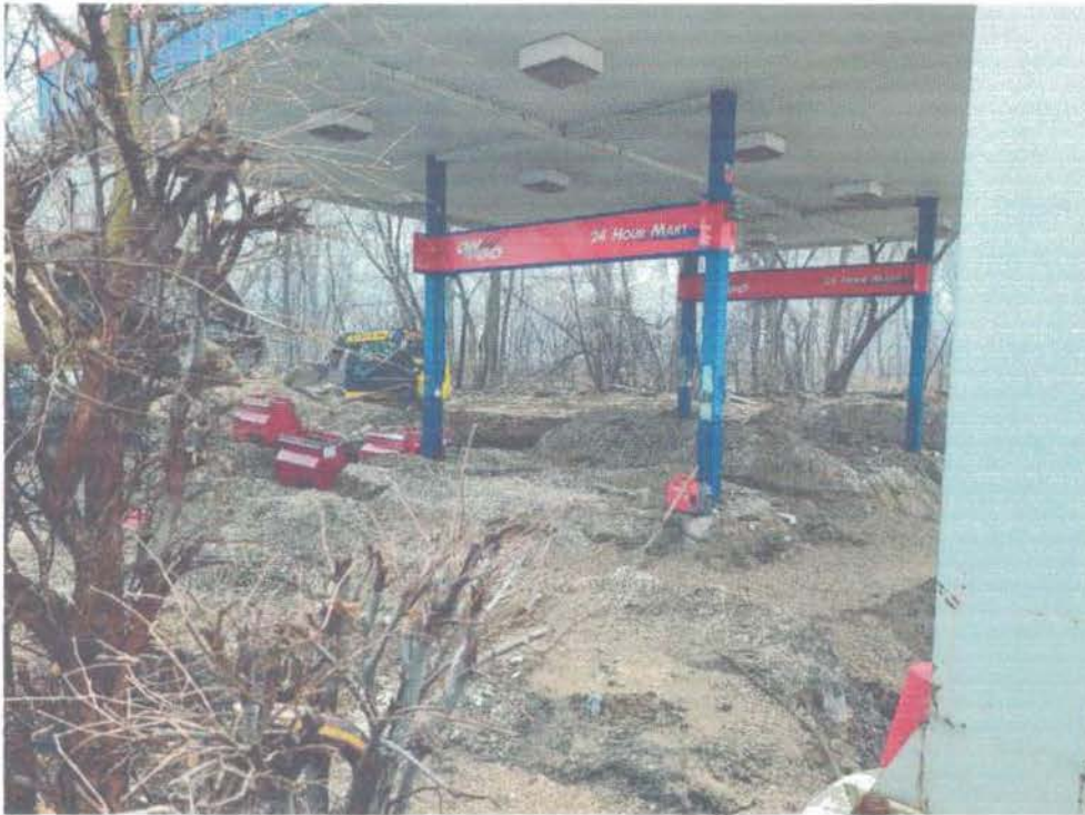
PHOTOGRAPH OF THE FORMER DISPENSER AREA
