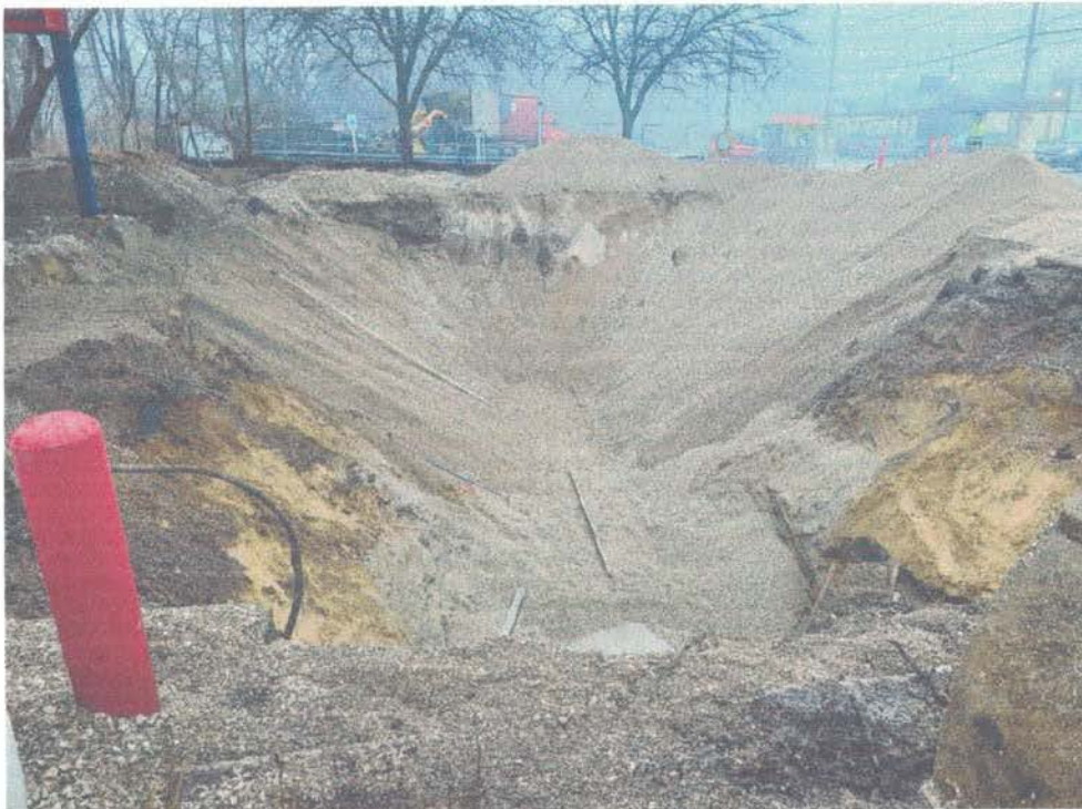
PHOTOGRAPH OF THE TANK BED AFTER OVER EXCAVATION
