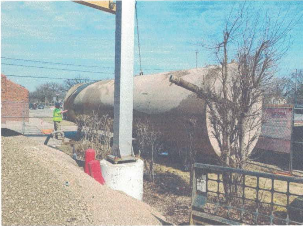
PHOTOGRAPH OF THE FIRST 12,000-GALLON TANK AFTER REMOVAL
