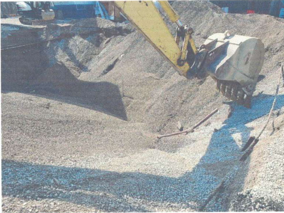
PHOTOGRAPH OF THE EXCAVATION AFTER REMOVAL OF TANKS
