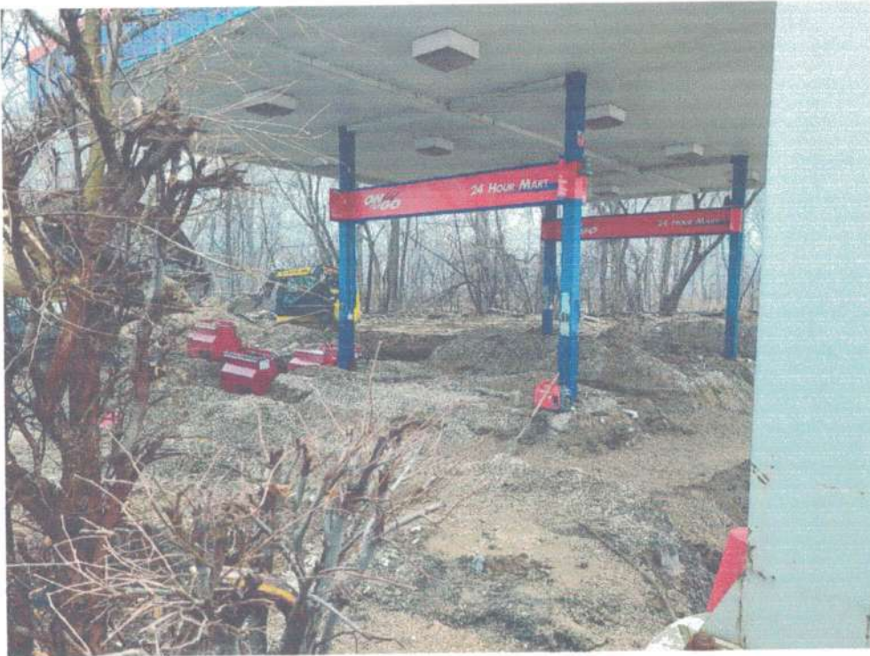
PHOTOGRAPH OF THE FORMER DISPENSER AREA
