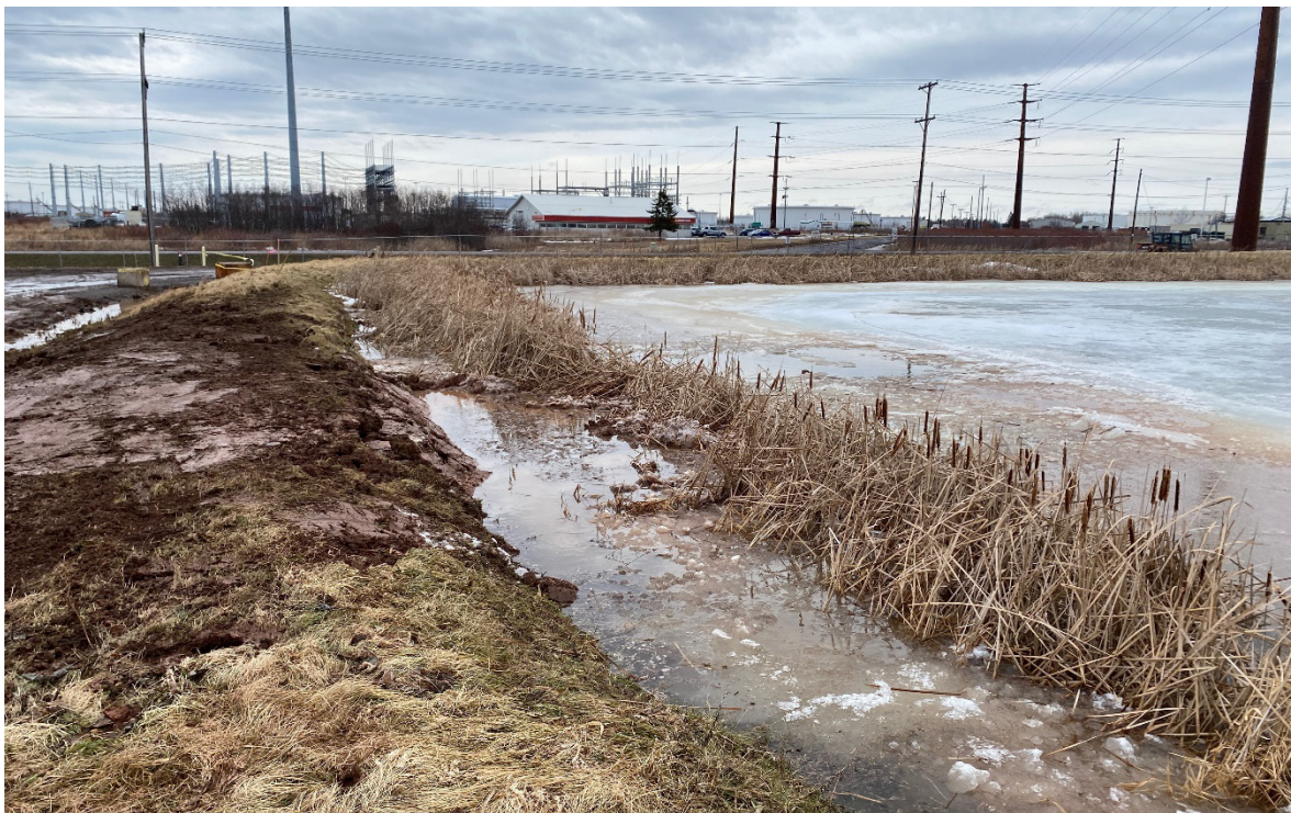
Photo 2 View of Stormwater Pond 4; non-vegetated area was location of hole from a muskrat in berm. Photo taken facing southeast on March 21, 2022.
