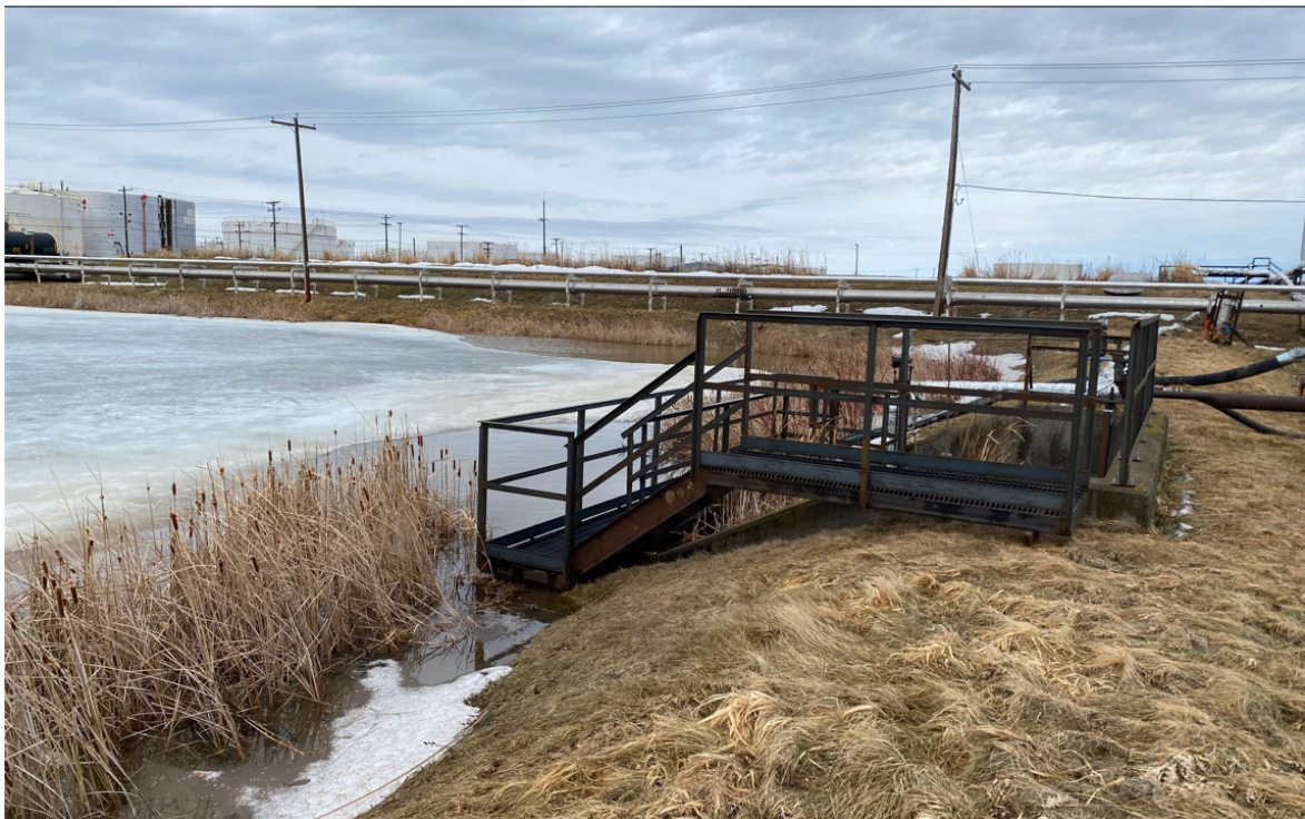
Photo 4 View of pond water sample platform. Platform is located near the northeast corner of the pond. Photo taken on March 21, 2022.
