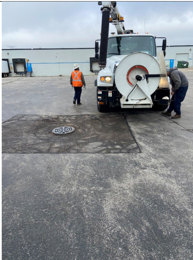
Photo 10: Jetting and vacuuming operation.
