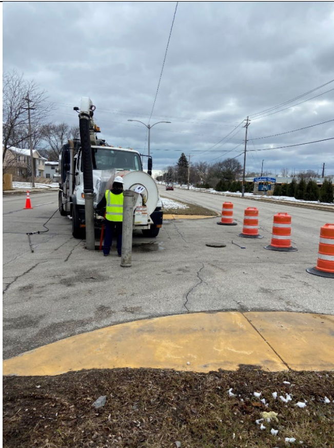
Photo 12: Jetting and vacuuming operation.
