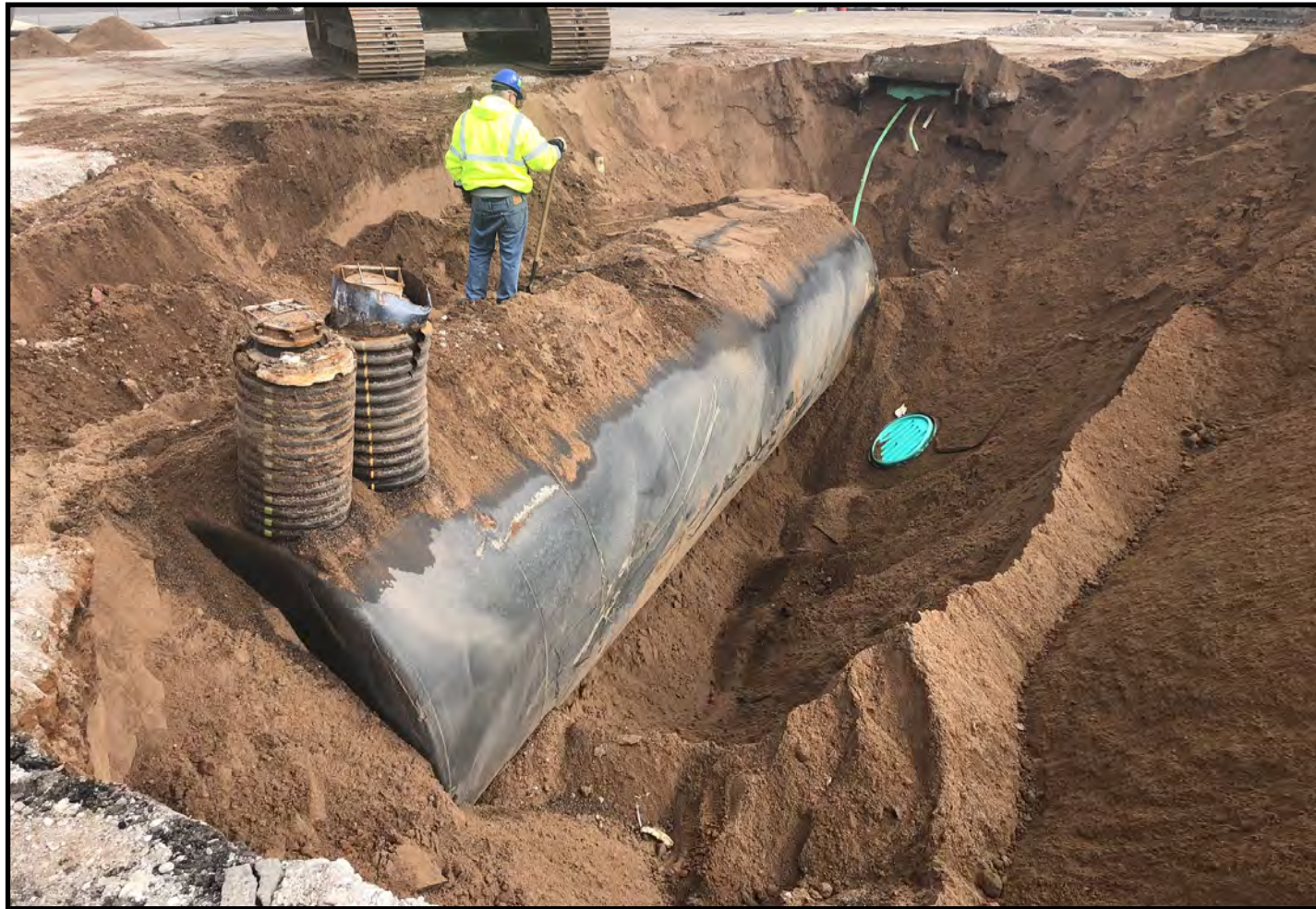
Removal of western tank.
