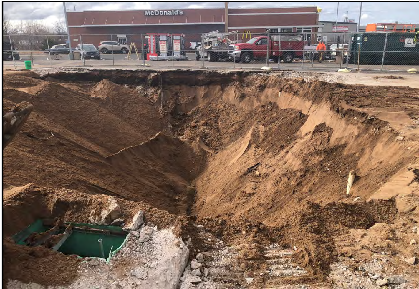
Tank bed upon removal of all USTs.
