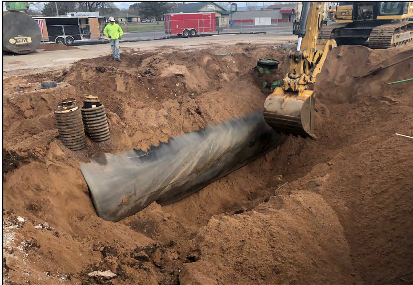
Removal of central tank, eastern tank previously removed.
