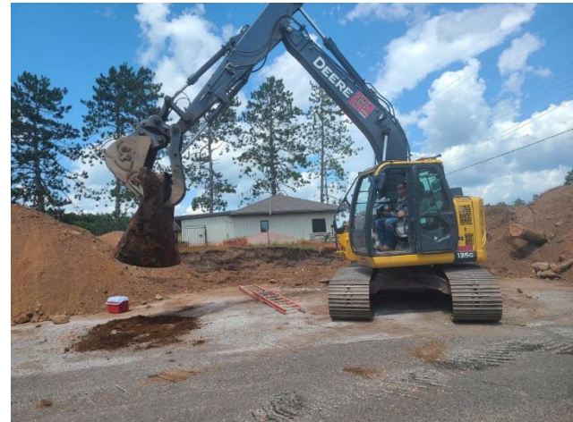
Additional view of tank after removal from basin.
