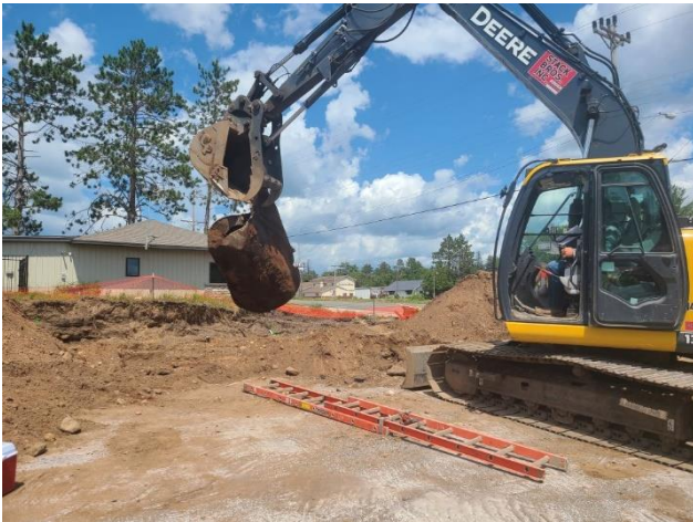
View of tank after removal from basin.
