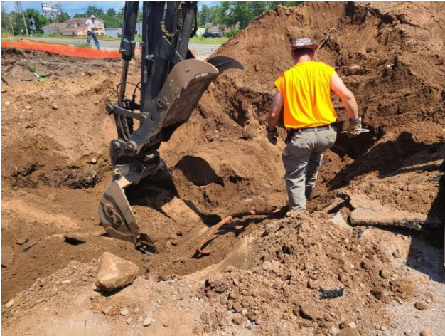
View of tank basin during removal activities.
