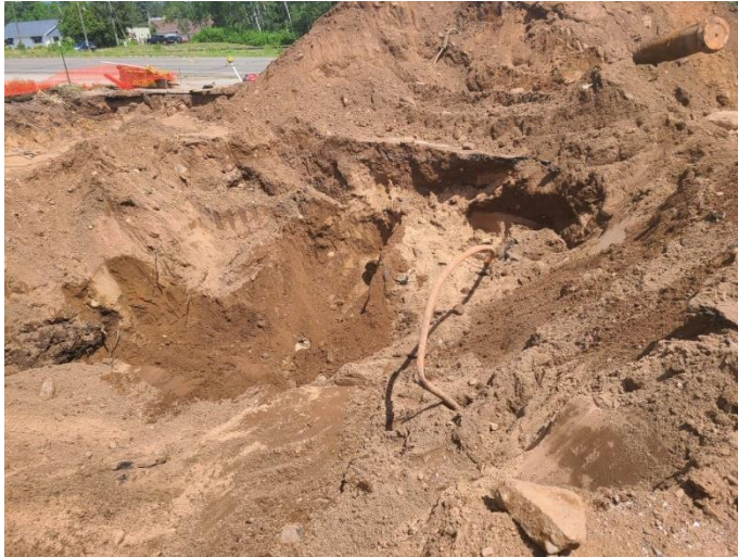
View of excavation after tank removal was completed.
