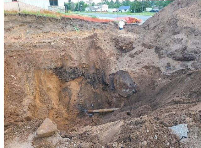
View of exposed tank after excavation.
