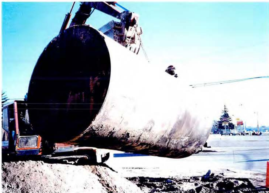
PHOTO 4 View of the 4,000 gallon gasoline tank being removed Tank 1.
