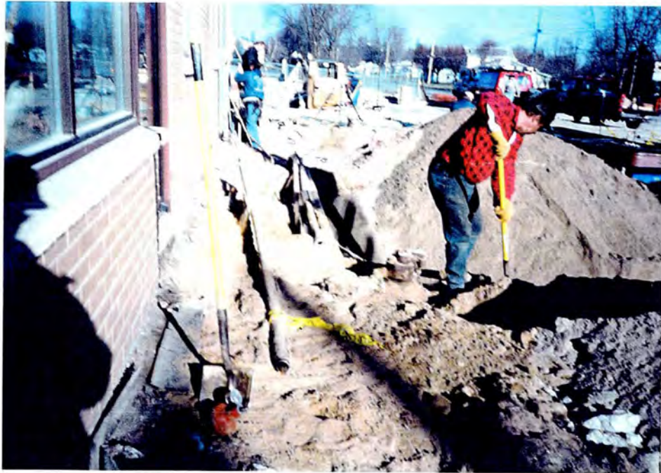
PHOTO 1 View of the product and vent piping along the east side of the building.
