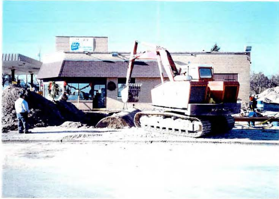
PHOTO 5 View of the 8,000 gallon gasoline tank being removed. Tank 2.
