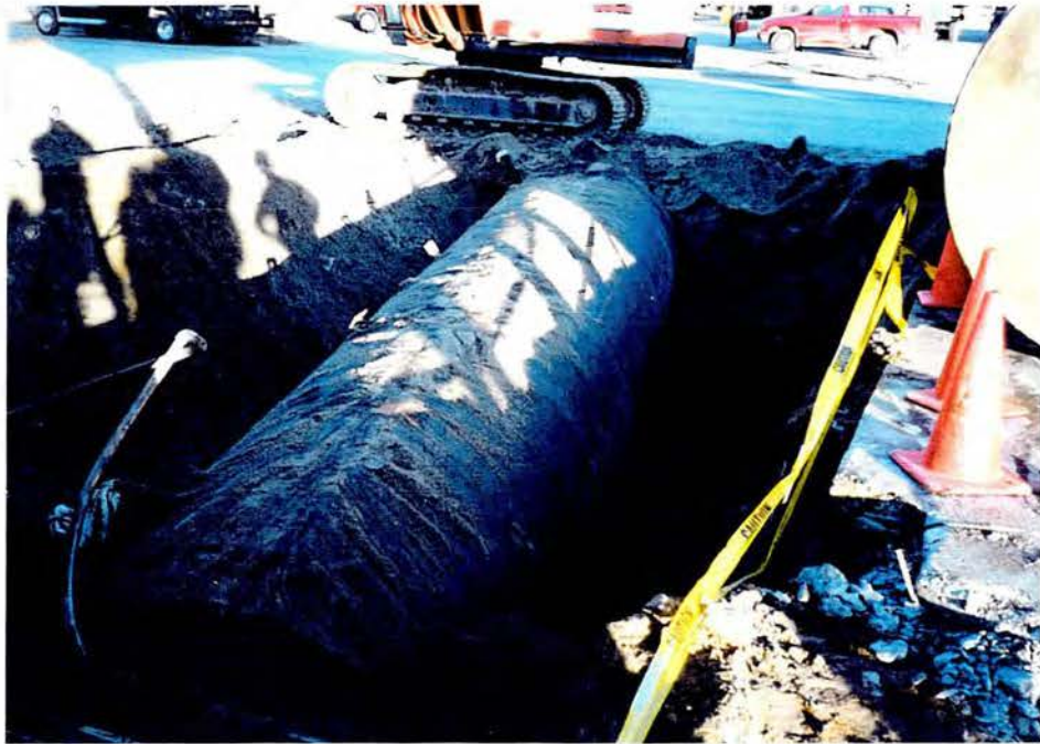
PHOTO 7 View of the 8,000 gallon diesel fuel tank prior to removal.
