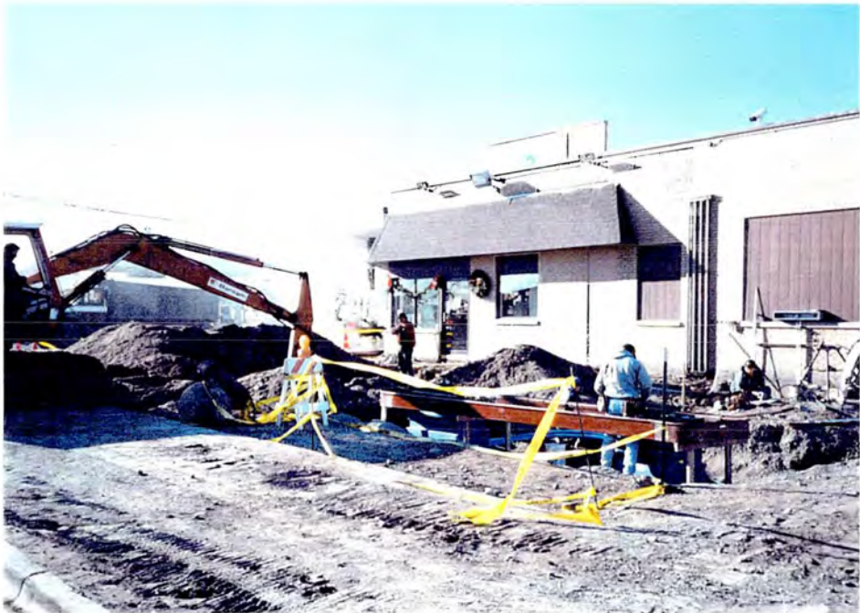
PHOTO 2 View of the former dispenser island area. New island being installed.
