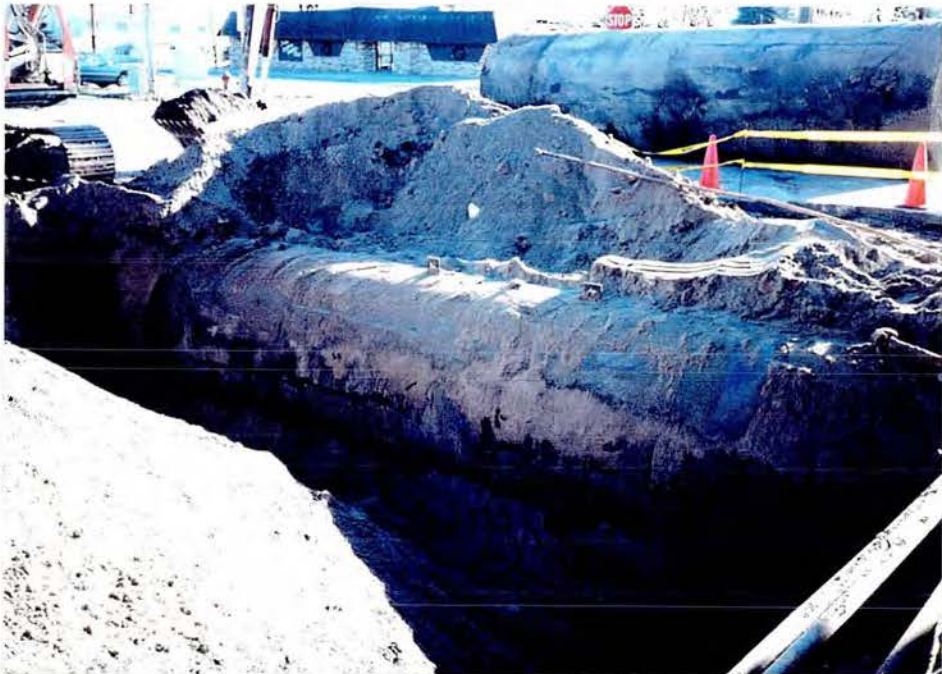
PHOTO 6 View of the excavation for the 8,000 gallon gasoline tank. Tank 3.
