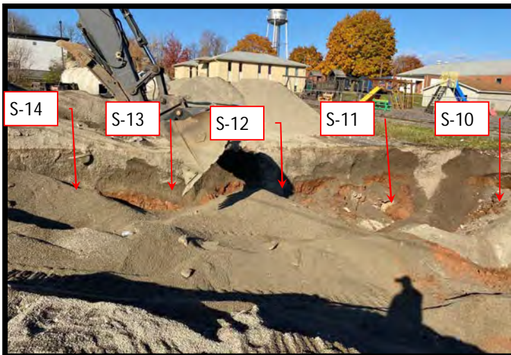
View West - W sidewall of excavation & soil samples S-10 through S-14.
