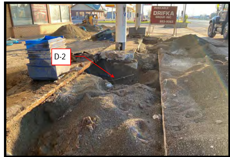
View East - Location of removed dispenser and sample D-2.
