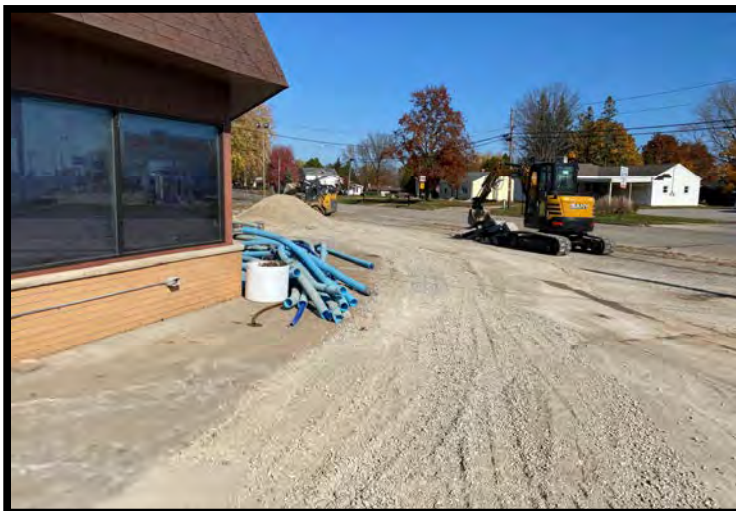
View Northeast - Overview of site upon completion of TSSA.
