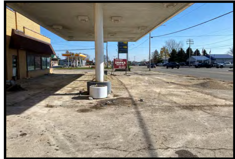
View East - Overview of site upon completion of TSSA.
