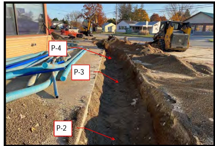
View Northeast - Location of piping run & soil samples P-2, P-3 & P-4.
