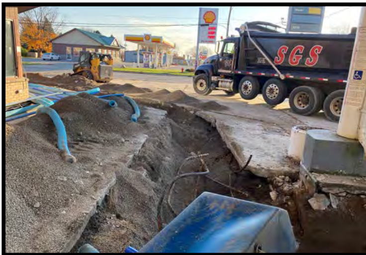
View East - Location of piping run.
