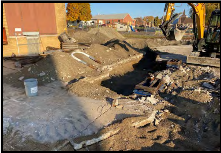
View Northwest - Overview of removed dispensers.
