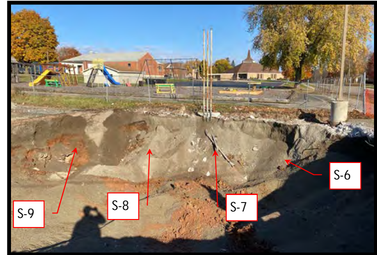
View North - N sidewall of excavation & soil samples S-6 through S-9.
