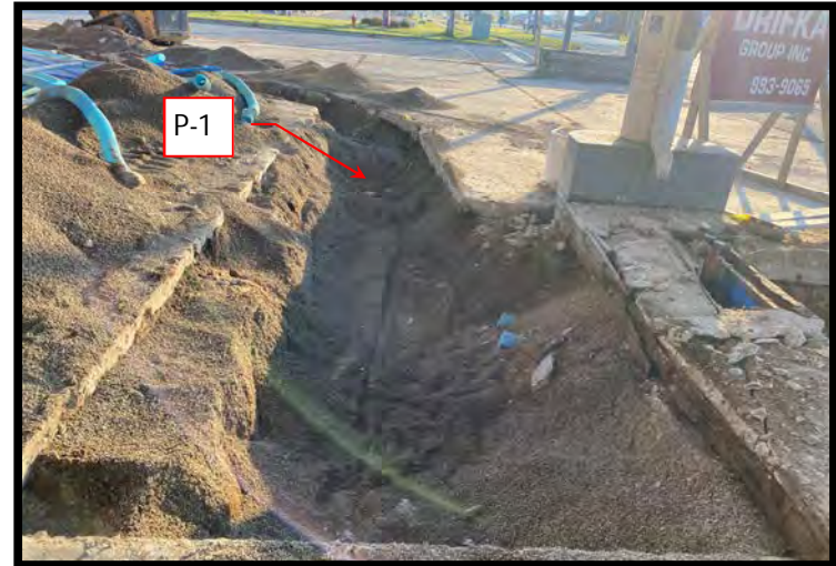
View East - Location of piping run and soil sample P-1.
