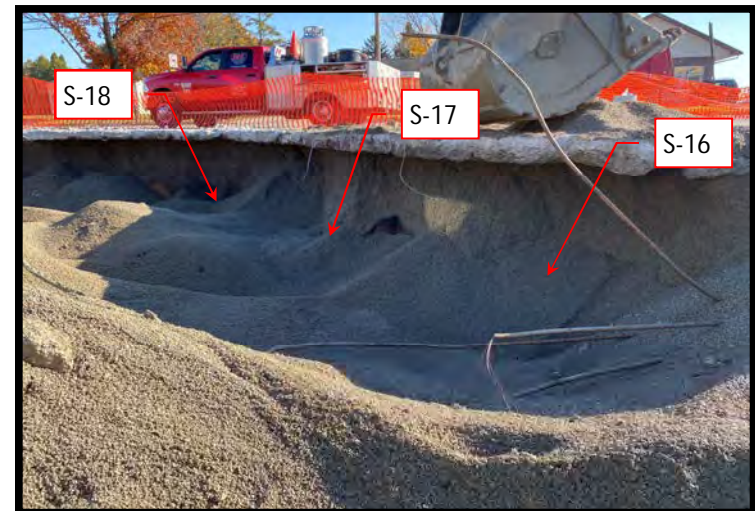
View East - S sidewall of excavation & soil samples S-16 through S-18.
