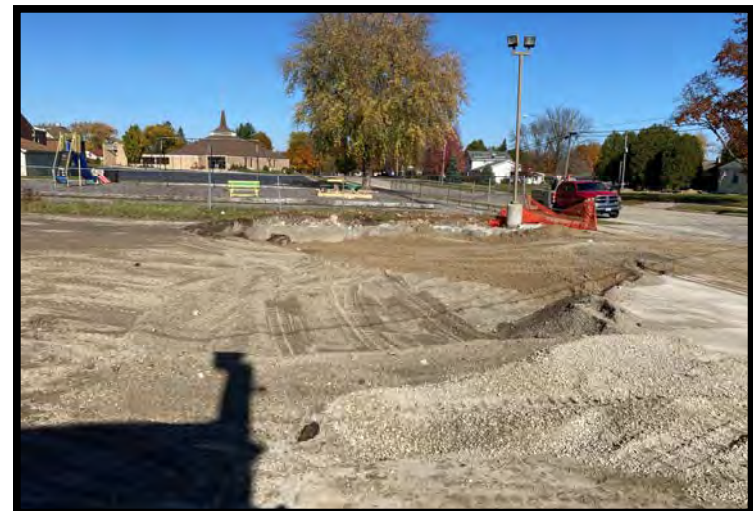
View North - Backfilling of tank excavation area upon completion of sampling.
