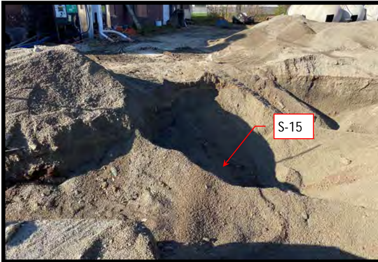
View West - S sidewall of the excavation & soil sample S-15.
