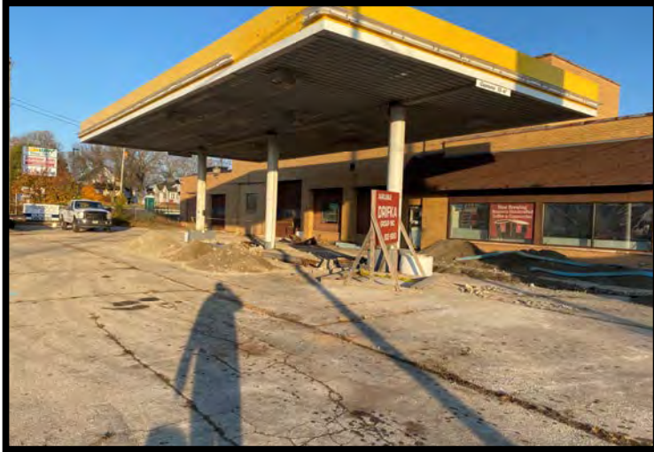
View Northwest - Overview of canopy and dispensers.
