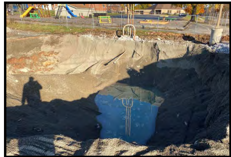
View North - Overview of tank bed & water in bottom of excavation.
