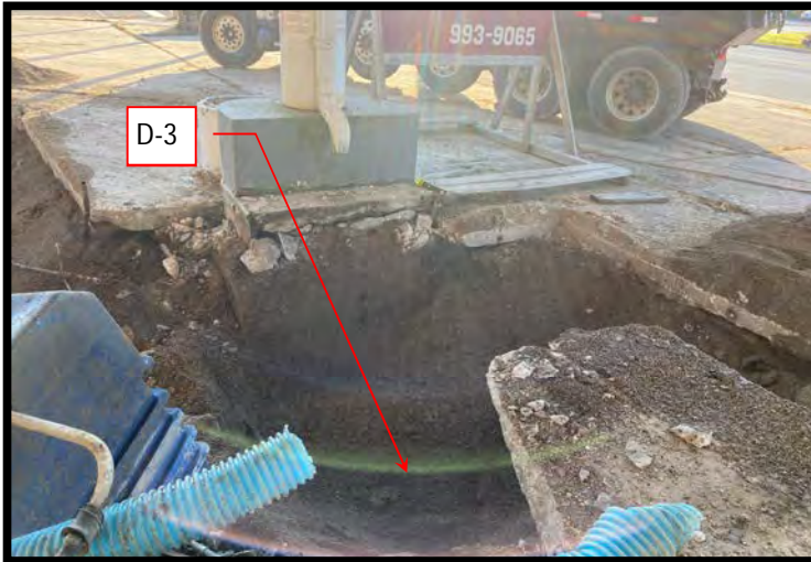
View East - Location of removed dispenser and sample D-3.
