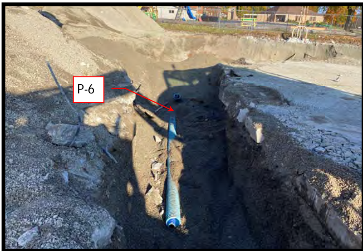
View North - Location of piping run and soil sample P-6.
