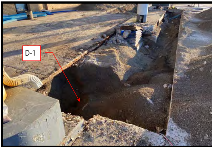
View East - Location of removed dispenser and sample D-1.
