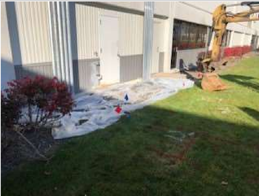
Photo # 3 : Close up view of plastic covering grass/landscape gravel in release area immediately adjacent to building
