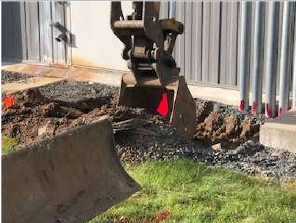
Photo # 4: Start of excavation activities
