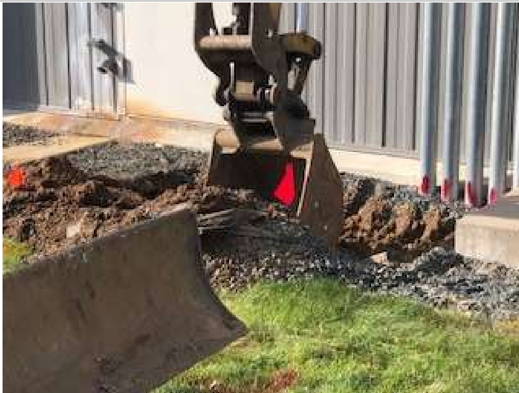
Photo # 4: Start of excavation activities
