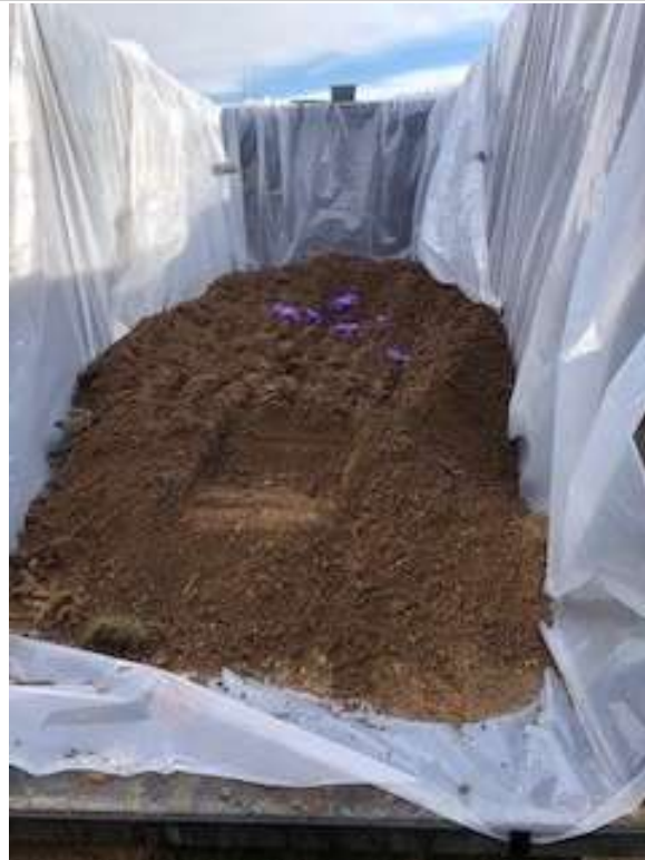
Photo # : Impacted grass, landscape gravel and sand in roll-off. Approx. 7.5 cubic yards final volume.
