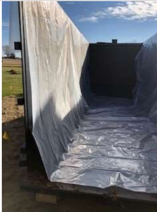
Photo # 5 : Plastic lining applied to new, unused, 40-yard roll-off container
