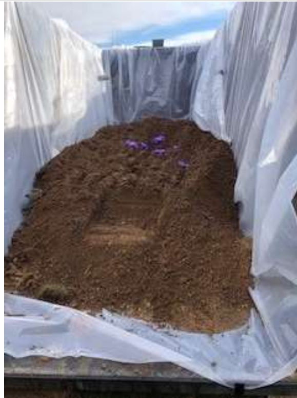
Photo # : Impacted grass, landscape gravel and sand in roll-off. Approx. 7.5 cubic yards final volume.
