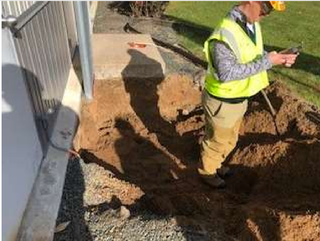
Photo # 6: Continuing with excavation of impacted grass and sand
