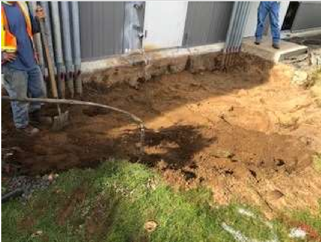
Photo # : Continuing with excavation of impacted grass and sand
