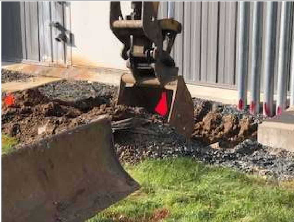
Photo # 4: Start of excavation activities
