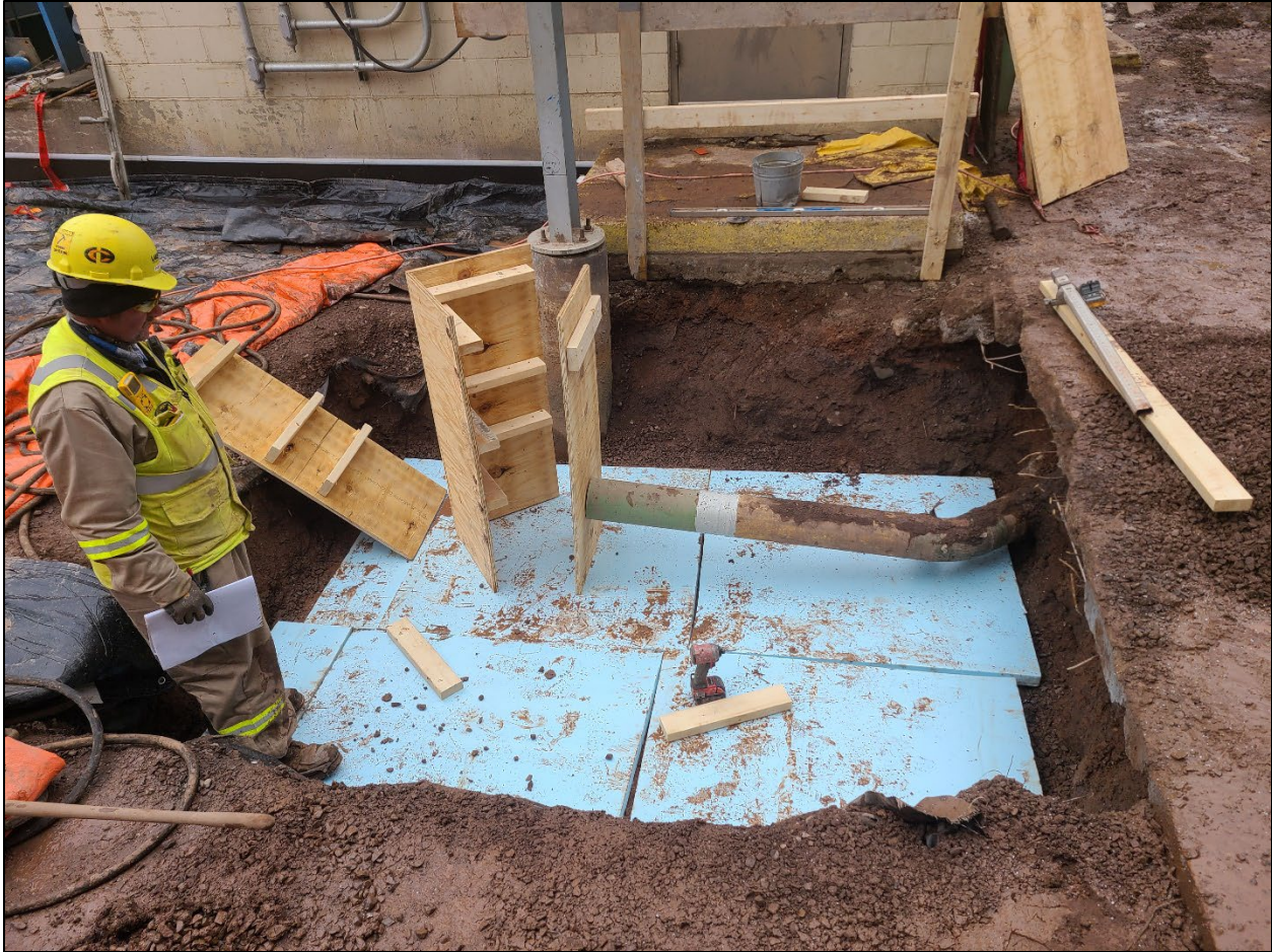
Photo 2 Excavation extent in Platformer Unit. Photo taken on December 7, 2022, by Insight.
