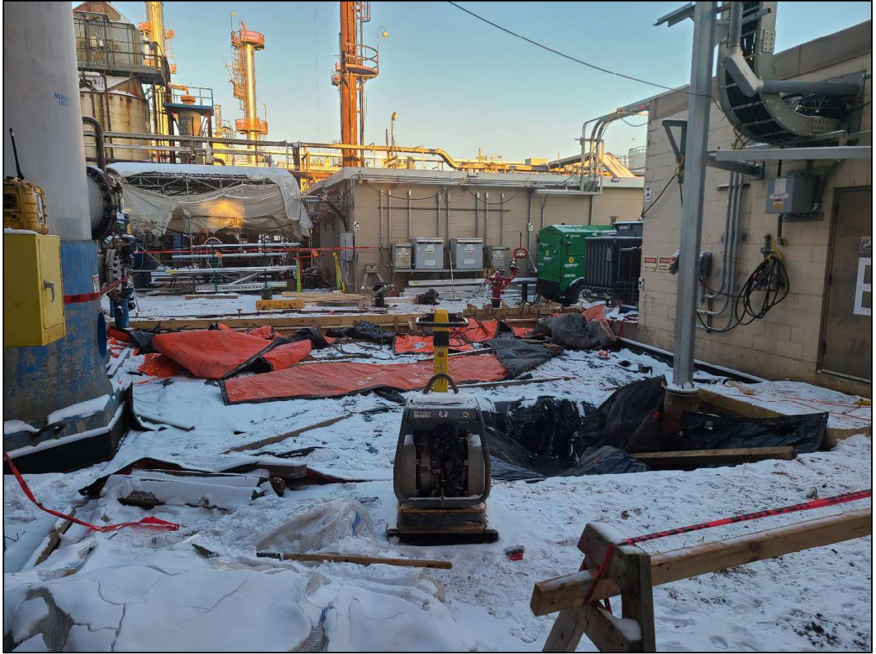
Photo 1 Excavation area in Platformer Unit. Photo taken on December 7, 2022, by Insight.
