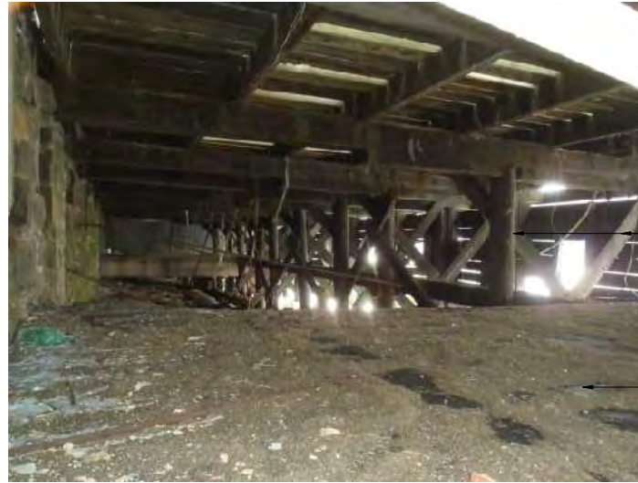
5 BENTS BELOW ELEVATED TIMBER DECK D502 / N.T.S.
