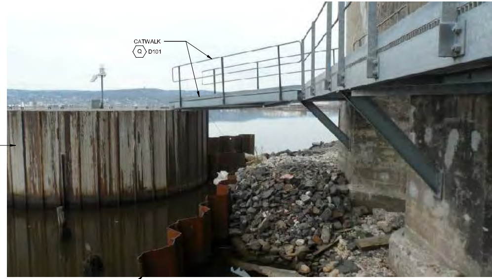
2 EXISTING PILES TO BE REMOVED D503 N.T.S.
