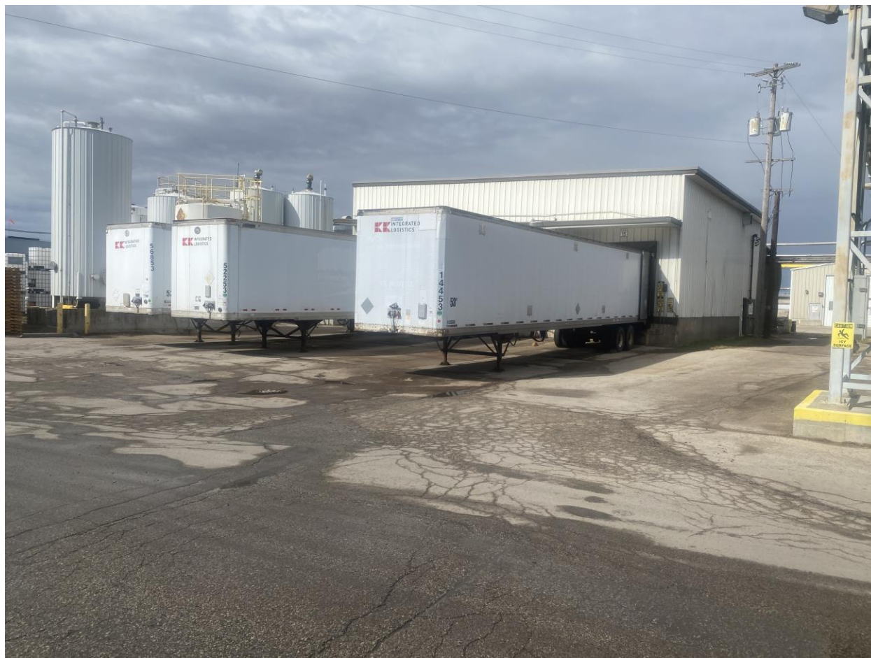
Photo of area after cleanup. Cleanup was completed before EHS personnel arrived to assess the spill.
