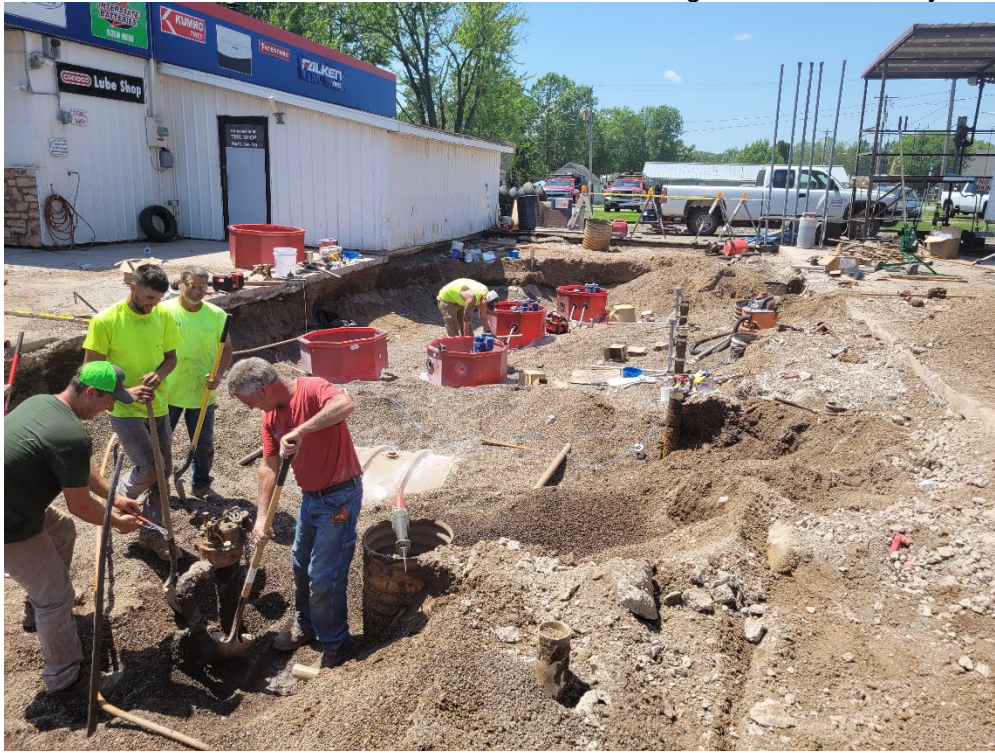
PHOTOGRAPH OF TRENCH OVER THE UST SYSTEM AND SUMP REPLACEMENT
