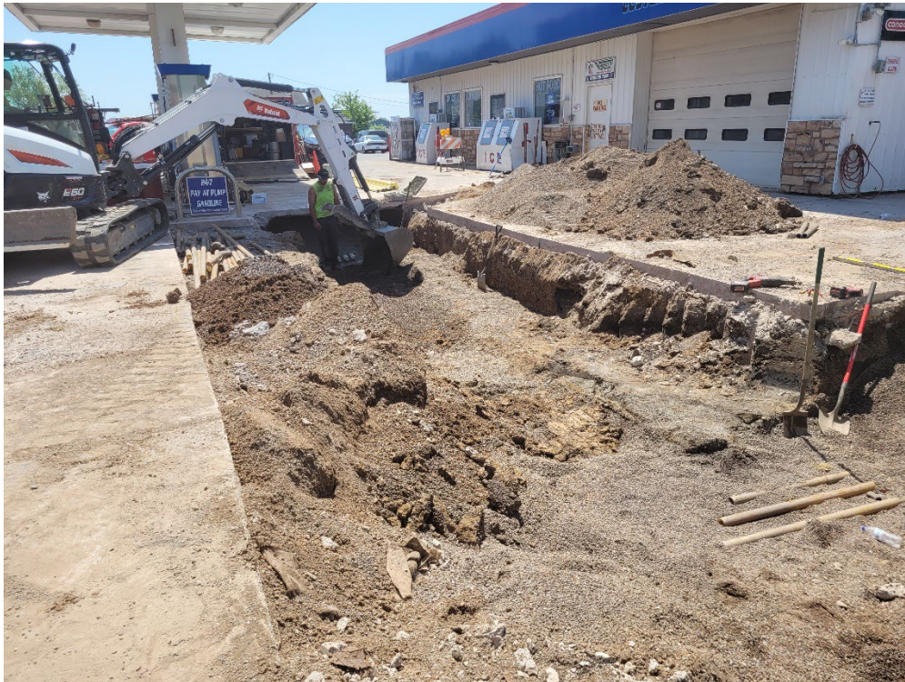
PHOTOGRAPH OF THE TRENCH VIEWING SOUTH TOWARDS THE DISPENSER ISLAND
