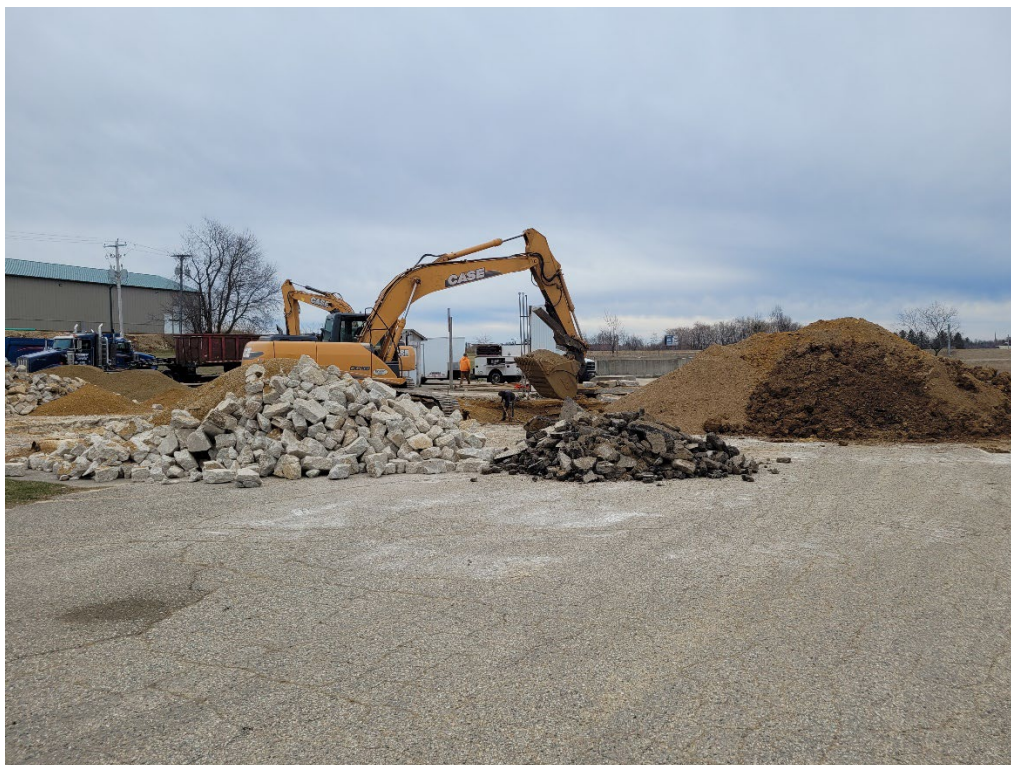
Photograph of the Site After Demolition of the Canopy
