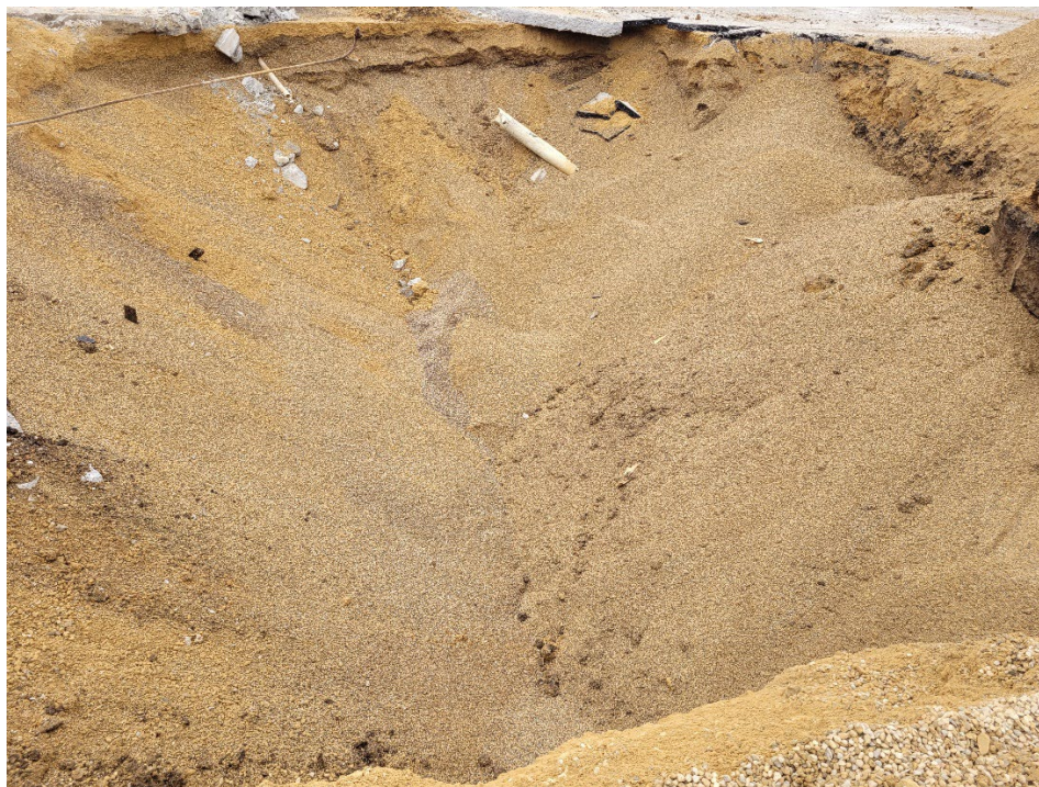
PHOTOGRAPH OF THE EXCAVATION AFTER REMOVAL OF THE 2 ND TANK
