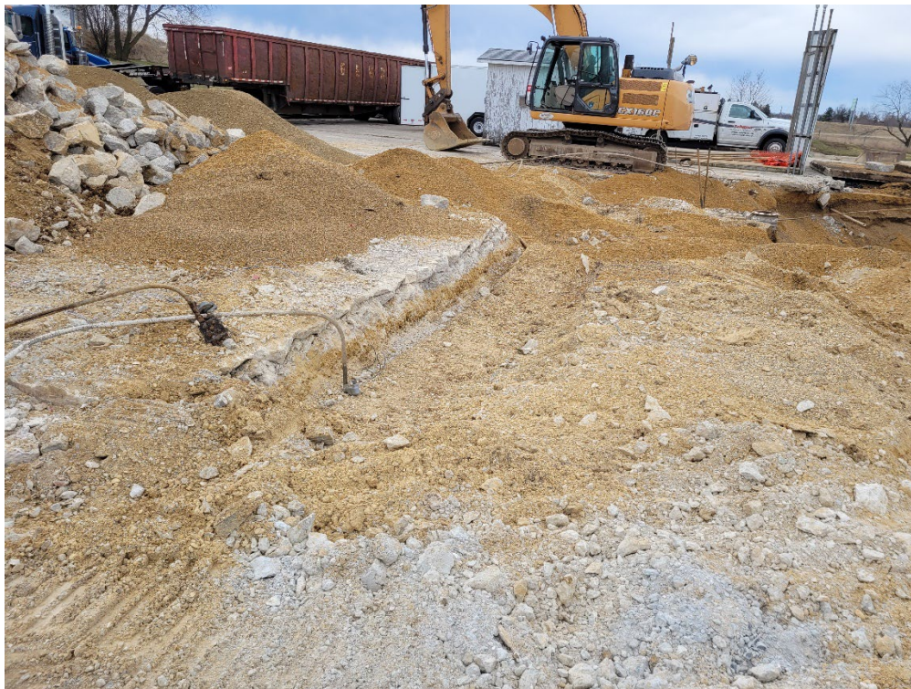
PHOTOGRAPH OF THE NORTHERN DISPENSERS AND PIPING
