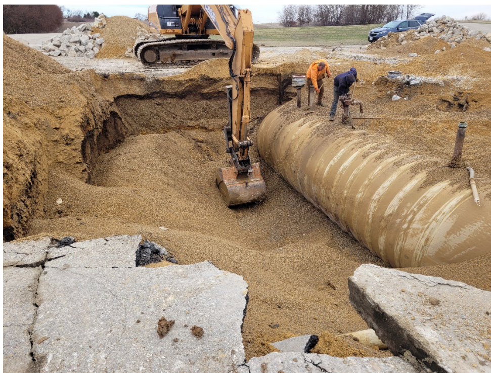
PHOTOGRAPH OF 2 ND UST REMOVED
