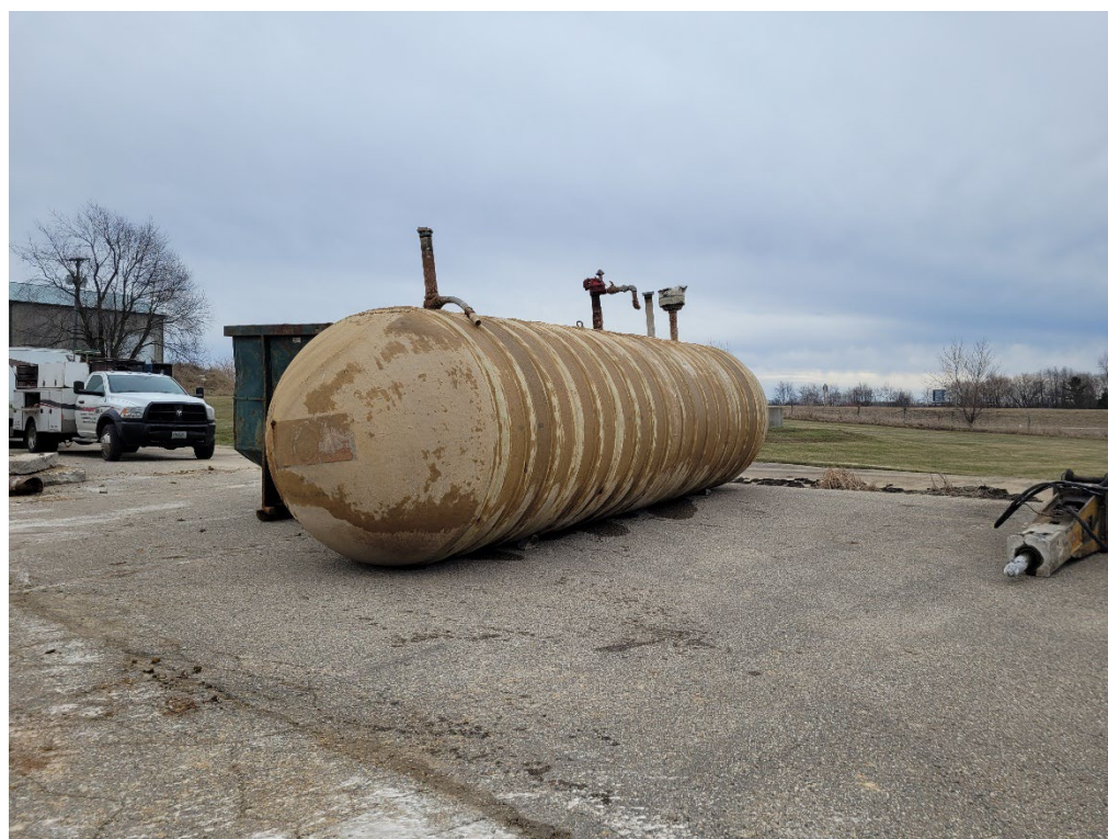
Photograph of 1 st Removed UST
