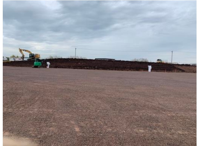
Light Pole Foundations & Berm Shaping
