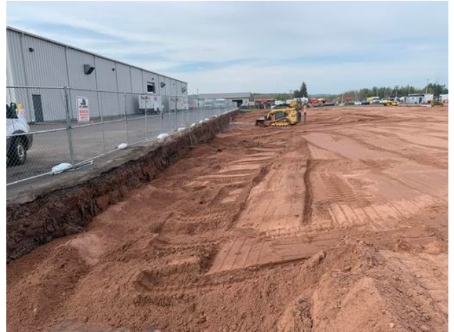
Sub-cut and import sand east lot transition
