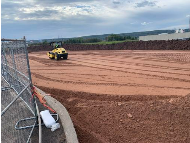
Compacting Sand on Trailer Lot
