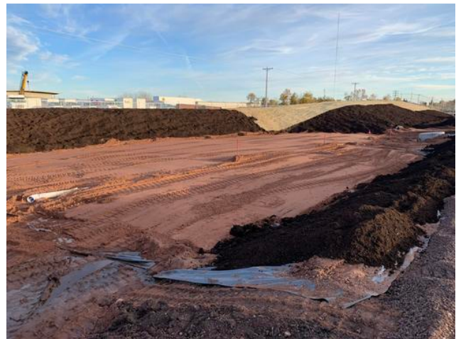
Topsoil, Draitile and Sand for Pond
