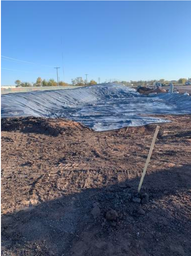
Pond & Berm PVC Liner
