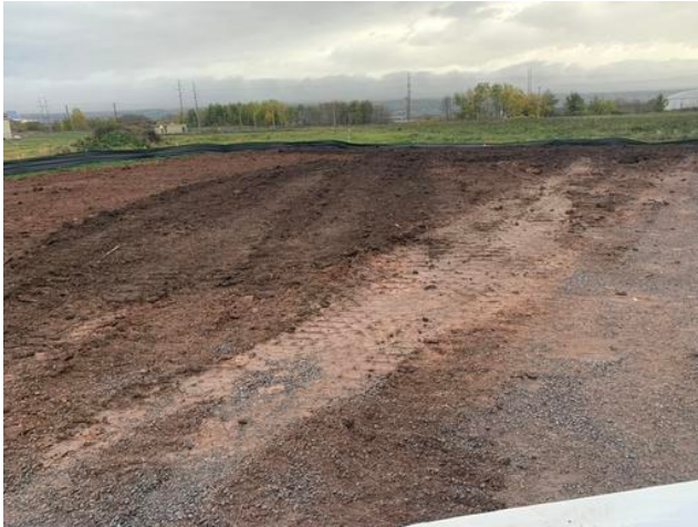
NW Site Perimeter Grading
