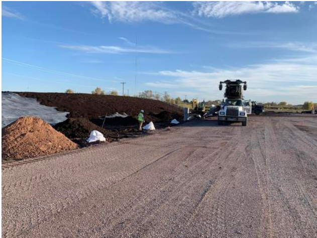
Berm Topsoil Placed by Conveyor
