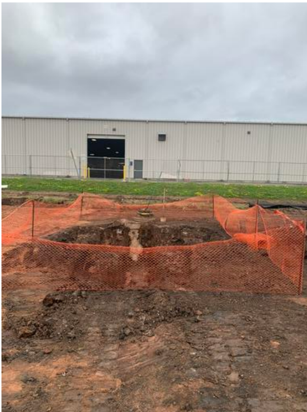
Catch Basin Tie-In Excavation
