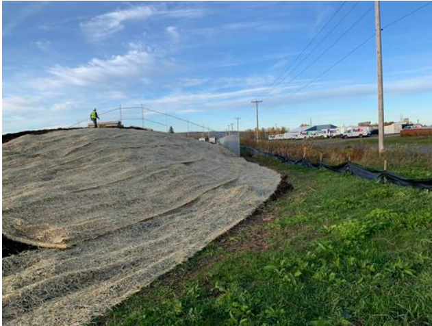
E-Mat @ SE Corner of Site
