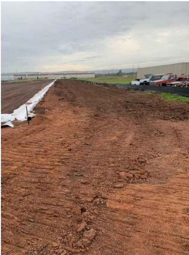
Grading North of Trailer Paving Curb
