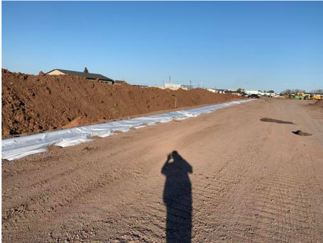
Trailer Curb Curing & Excavated Spoils
