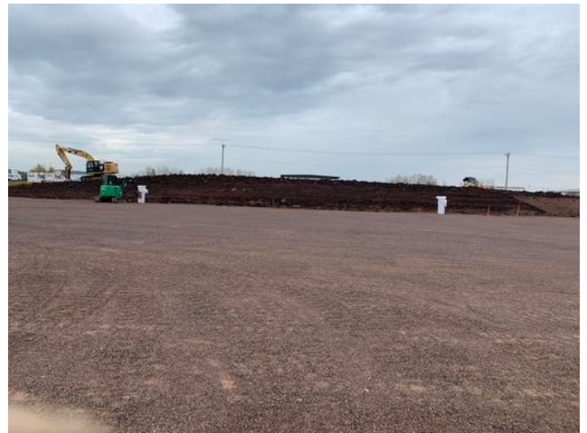
Light Pole Foundations & Berm Shaping
