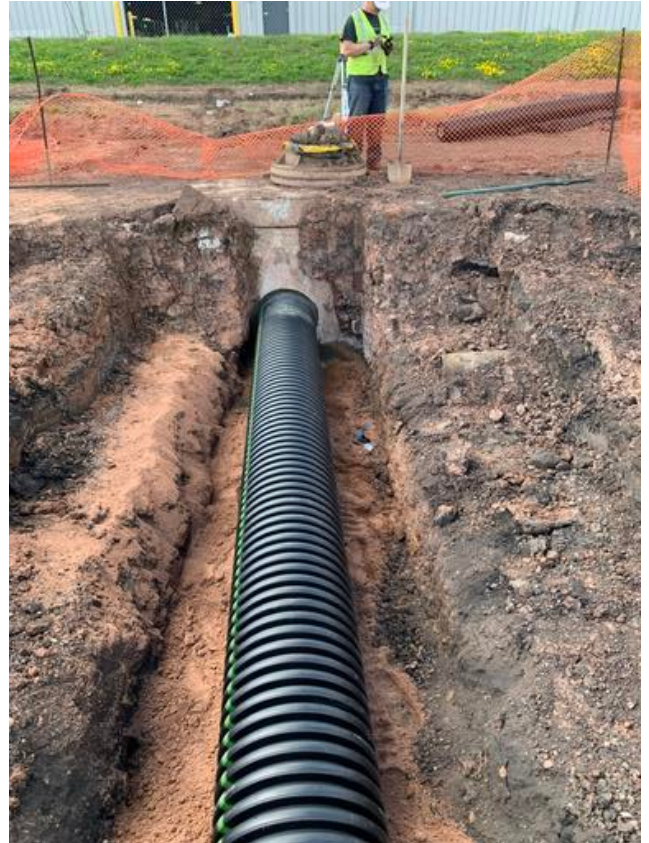
Catch basin tie-in
