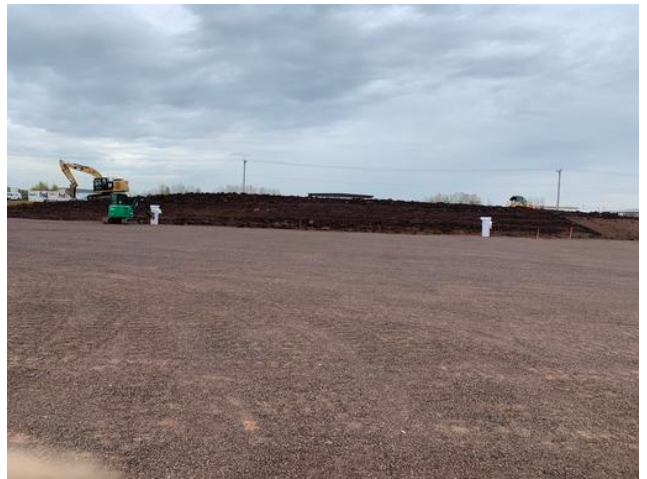
Light Pole Foundations & Berm Shaping
