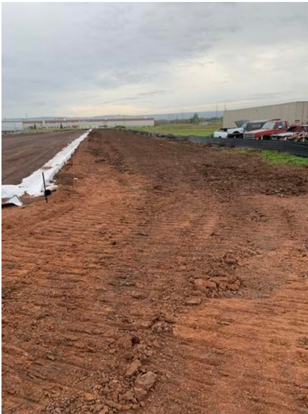
Grading North of Trailer Paving Curb
