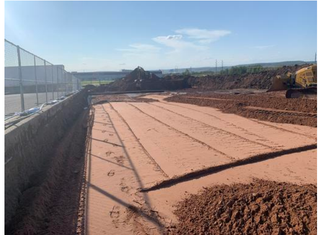
Fabric & Sand Placement @NW Trailer Lot
