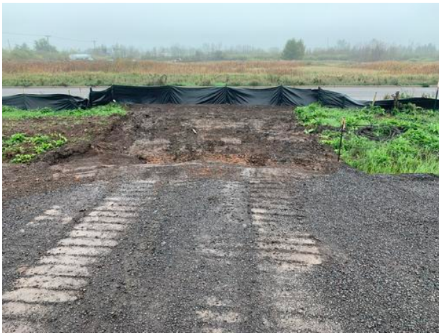
South Entrance Removed
