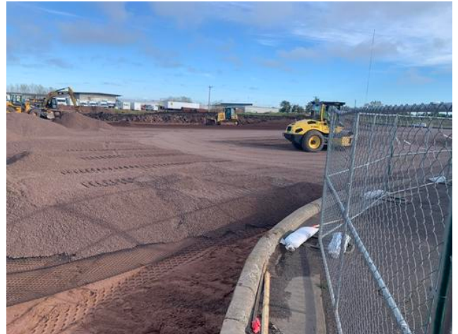
Geogrid, Gravel and Compaction at NE Corner of Lot
