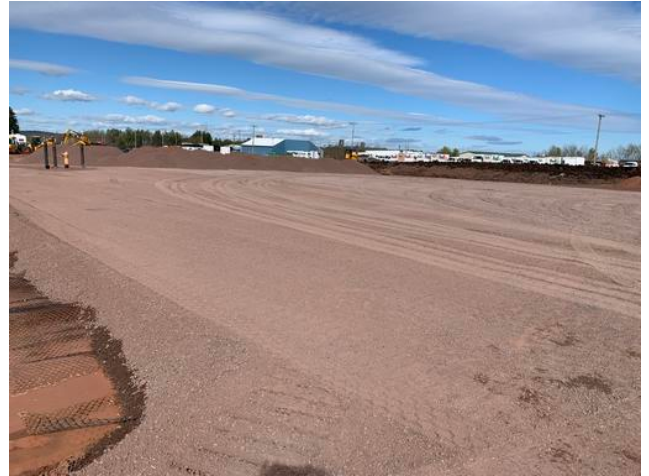
GeoGrid and Gravel on Van Lot
