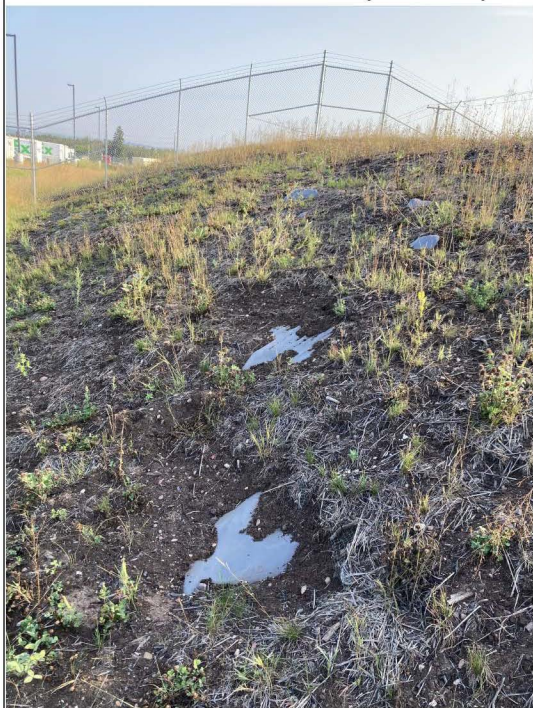
Title: Exposures of cap/liner material at southwest end of berm, viewing north.
