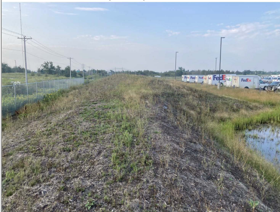
Title: Berm viewing south, storm water detention pond on right. Note scarce vegetation.
