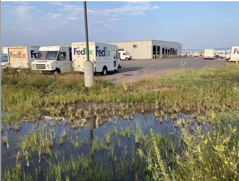
Title: North end of storm water pond viewing west. Note asphalt parking lot in background which also serves as cap/cover.
