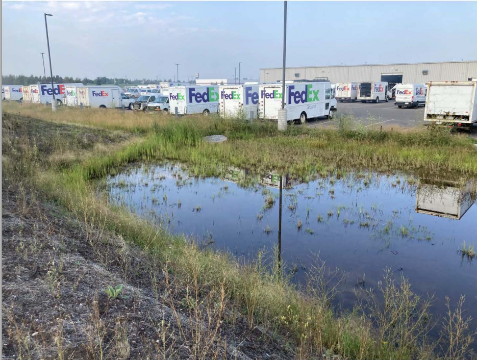
Title: South half of storm water pond viewing southwest. Note outflow structure in center at end of pond.
