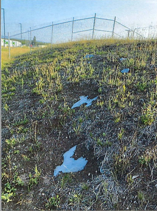
Title: Exposures of cap/liner material at southwest end of berm, viewing north.
