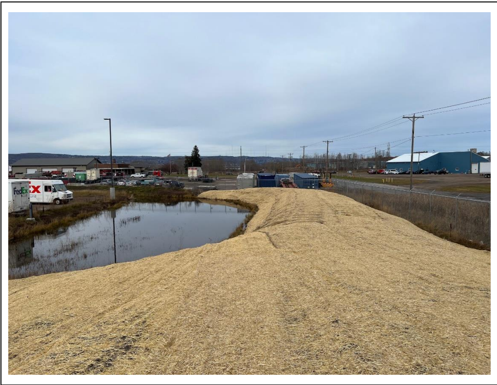
Photograph 7 - Soil Berm with seed mats
