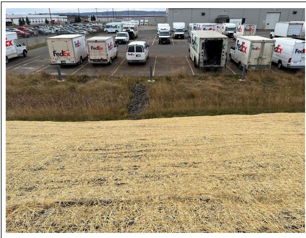
Photograph 4 - Soil Berm with seed mats
