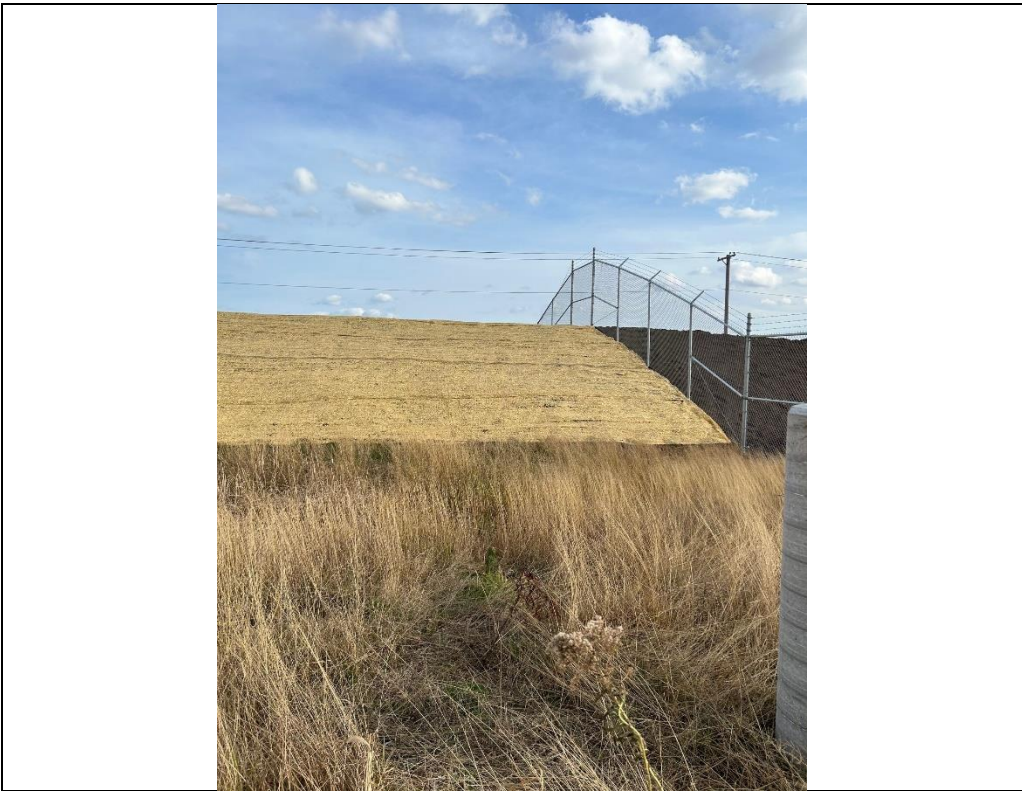
Photograph 6 - Soil Berm with seed mats
