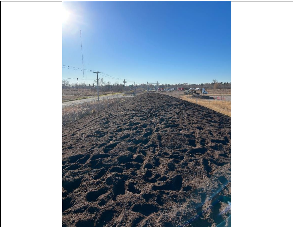
Photograph 9 - Soil cover on the berm
