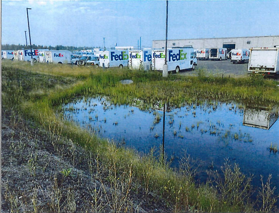
Title: South half of storm water pond viewing southwest. Note outflow structure in center at end of pond.
