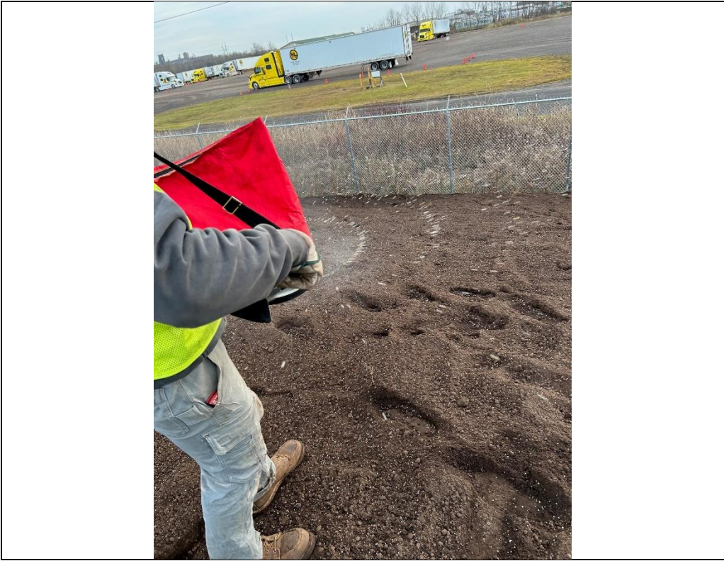
Photograph 8 - Dispersion of seed for grass coverage on berm.
