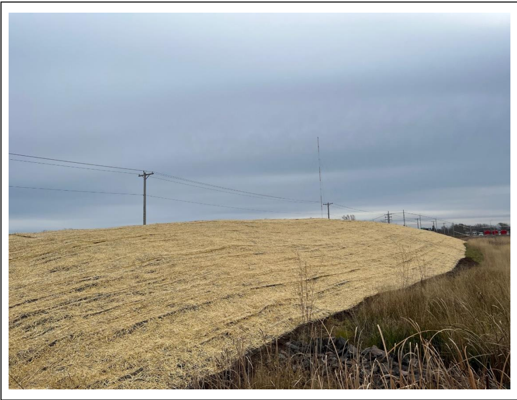
Photograph 5 - Soil Berm with seed mats
