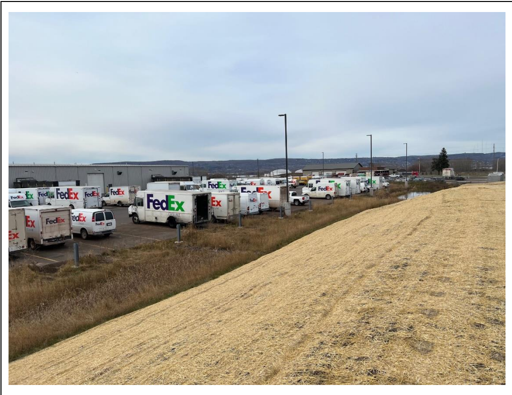
Photograph 2 - Soil Berm with seed mats
