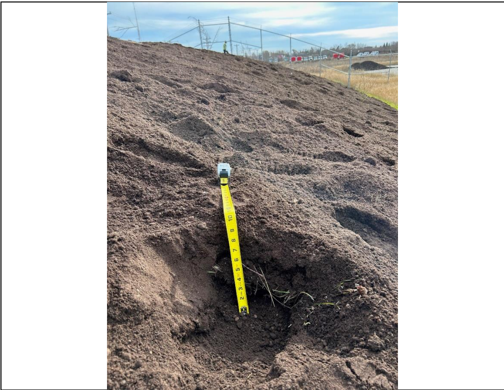
Photograph 10 - Showing Depth of Soil Coverage.
