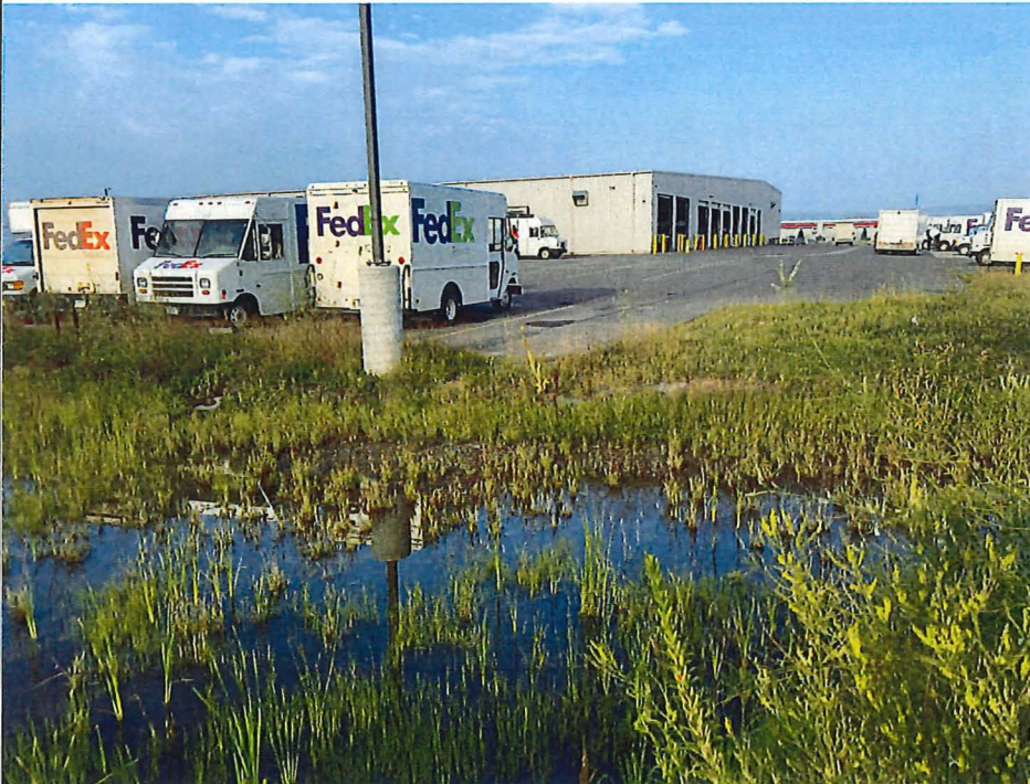
Title: North end of storm water pond viewing wes. Note asphalt parking lot in background which also serves as cap/cover.
