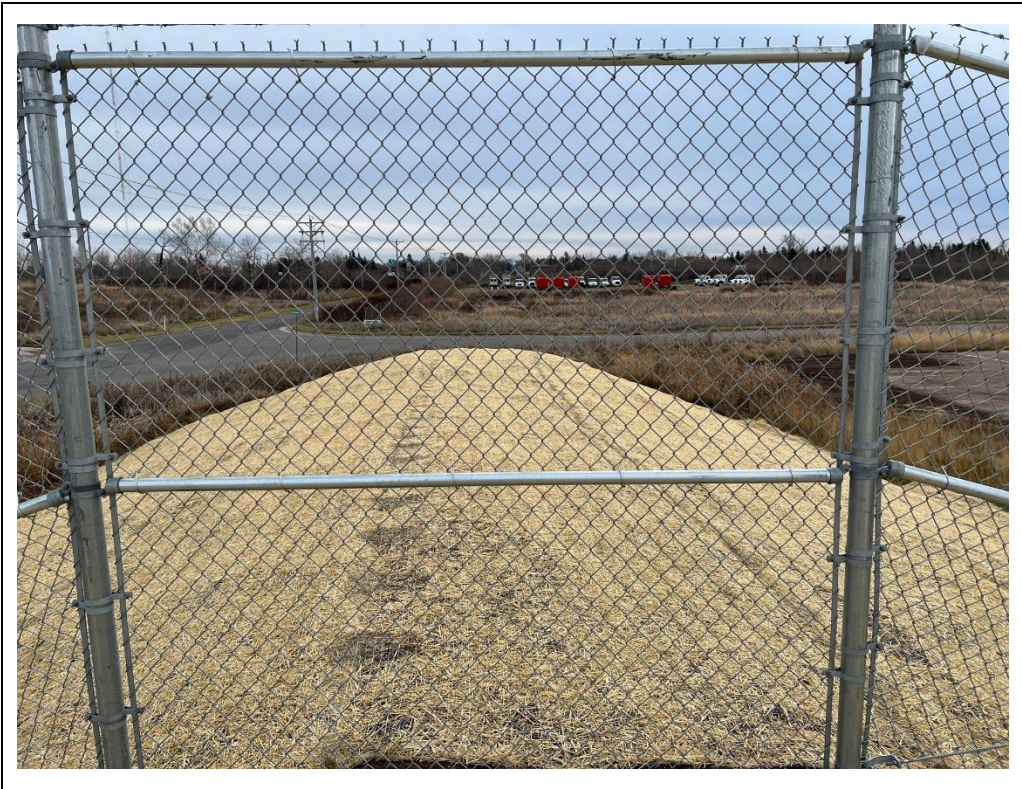
Photograph 1 - Soil Berm with seed mats
