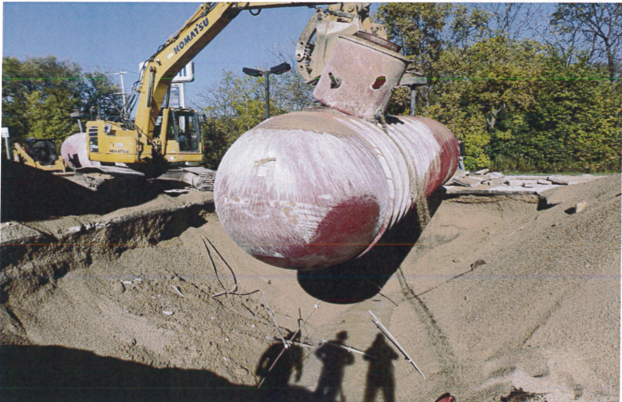
Photo 8 – Removal of northernmost UST from basin
