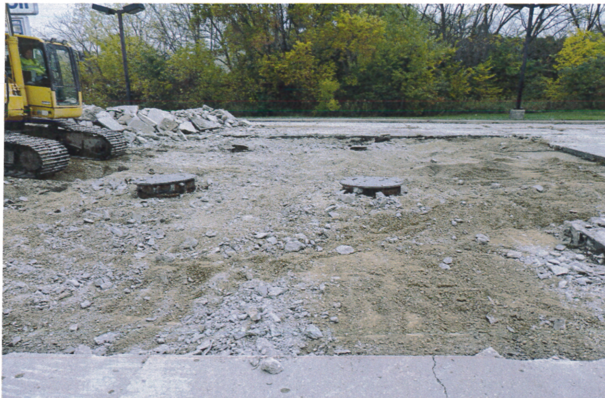
Photo 1 – View looking east/northeast across UST basin upon concrete removal
