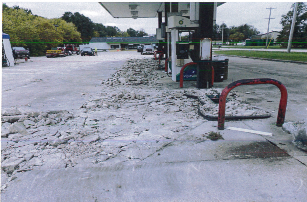
Photo 2 – View looking southwest from NE dispenser during concrete removal
