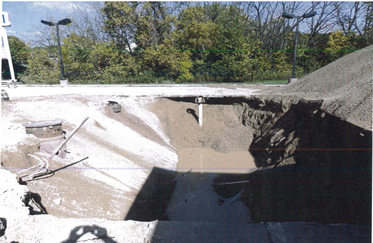
Photo 6 – View of basin upon removal of southernmost UST for cleaning
