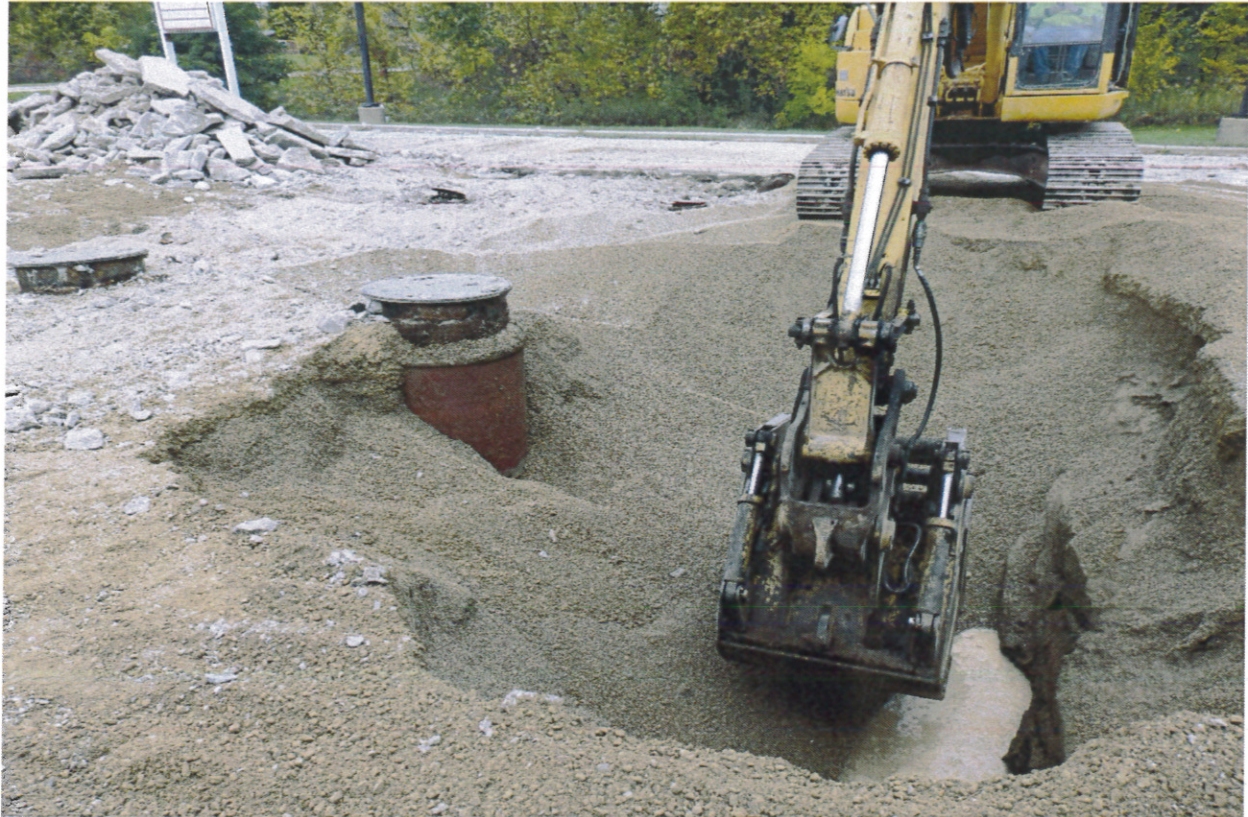
Photo 3 – Commencement of excavation alongside southernmost UST
