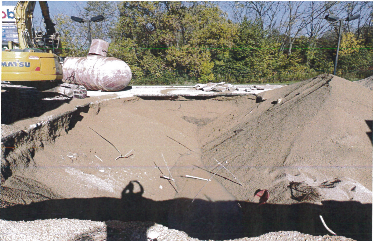
Photo 10 – View of UST basin with northernmost UST removed for cleaning
