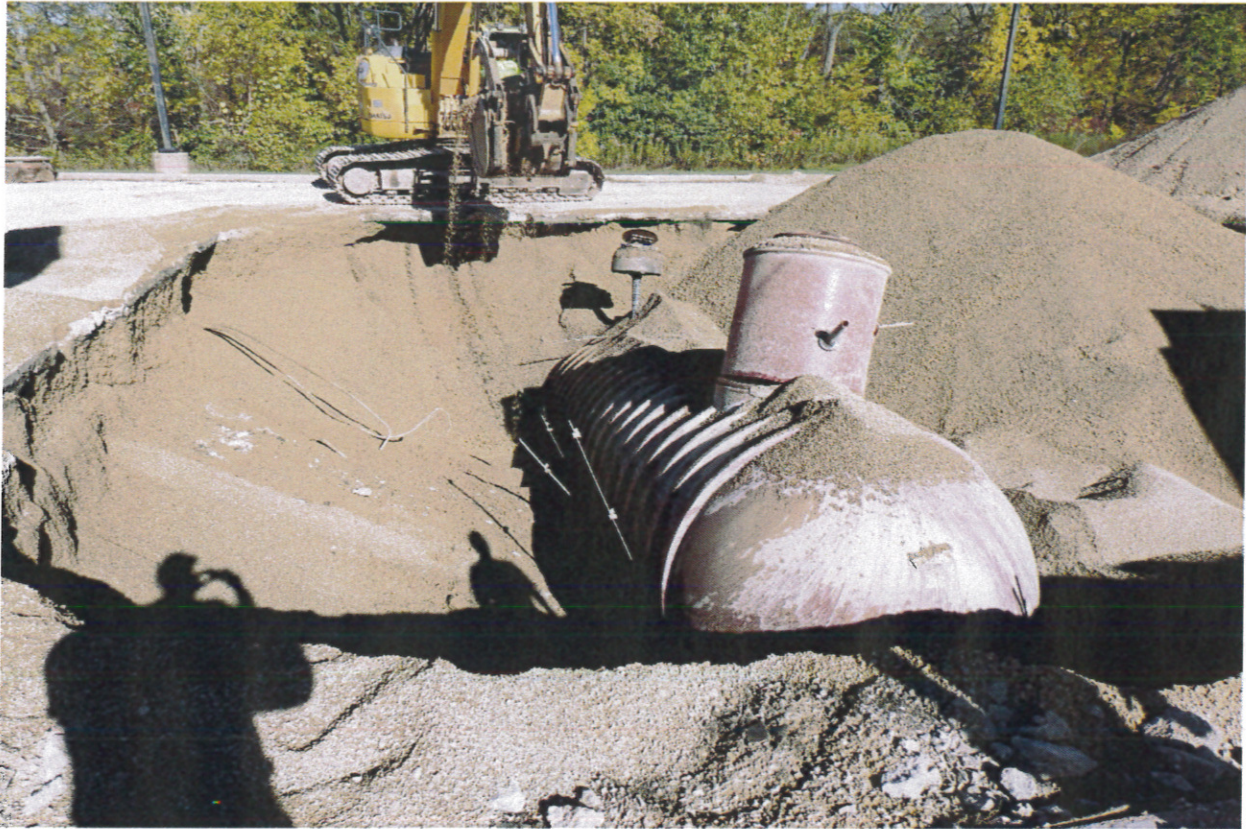
Photo 7 – Removal of northernmost UST
