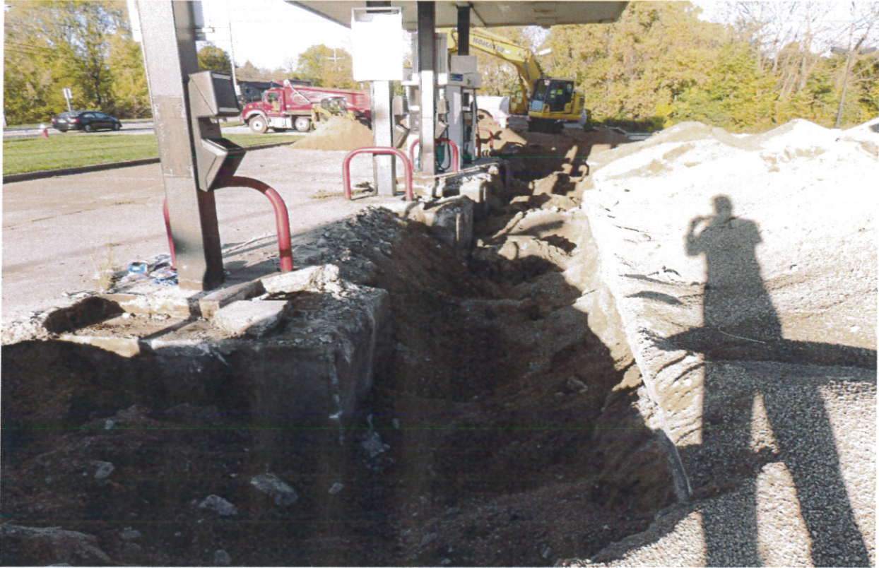
Photo 13 – View looking northeast from the SW dispenser along piping trench
