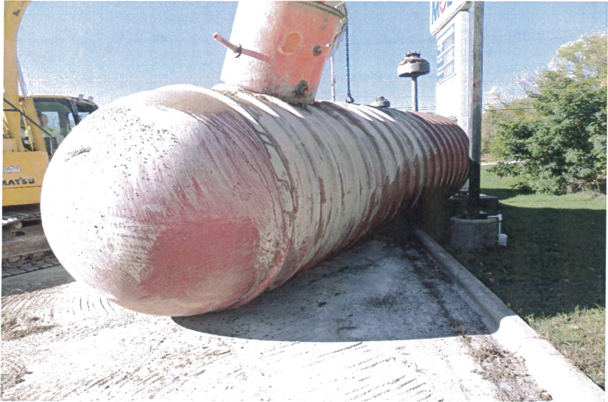
Photo 9 – View of second UST out of basin for cleaning
