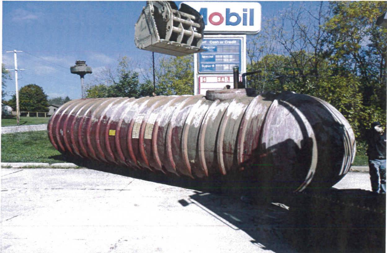
Photo 5 – View of southernmost UST out of basin for cleaning
