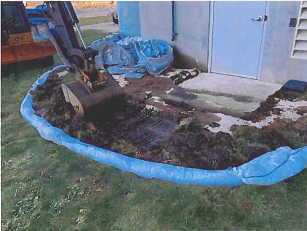
Mid-Project: Removing impacted soil with a mini-excavator.
