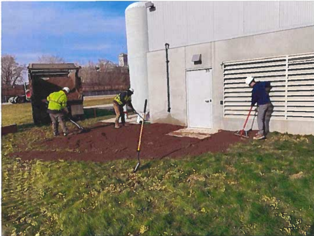
Mid-Project: Grading the backfilled topsoil following the excavation.
