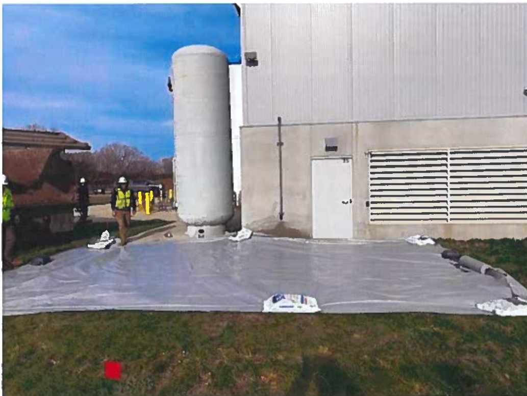
Post-Project: Covering the excavation area following the backfilling with topsoil.
