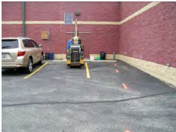
3. A view of boring B-1 on north side of building.
