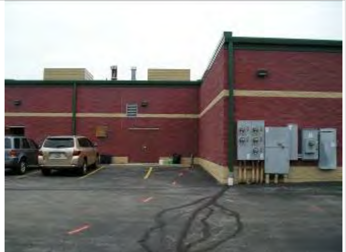
2. A view of the rear entrance to dry cleaners looking south.
