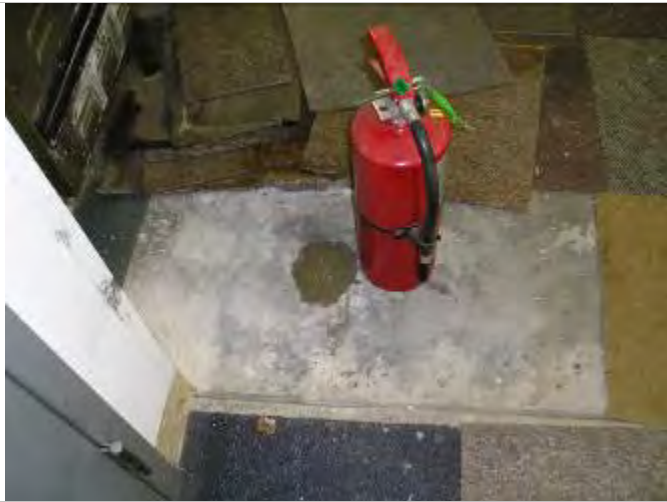
7. A view of boring B-2 patched with concrete.
