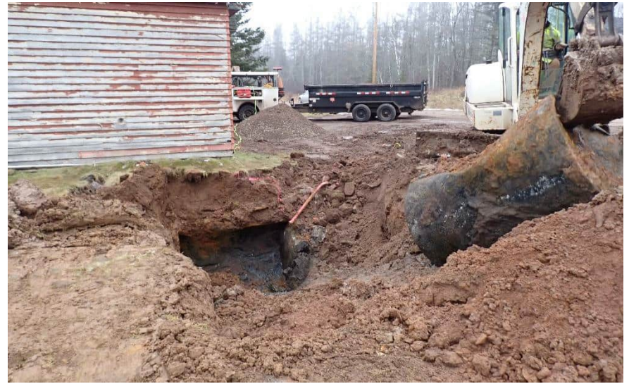
Removed 550-gallon tank and excavation area, facing west.
