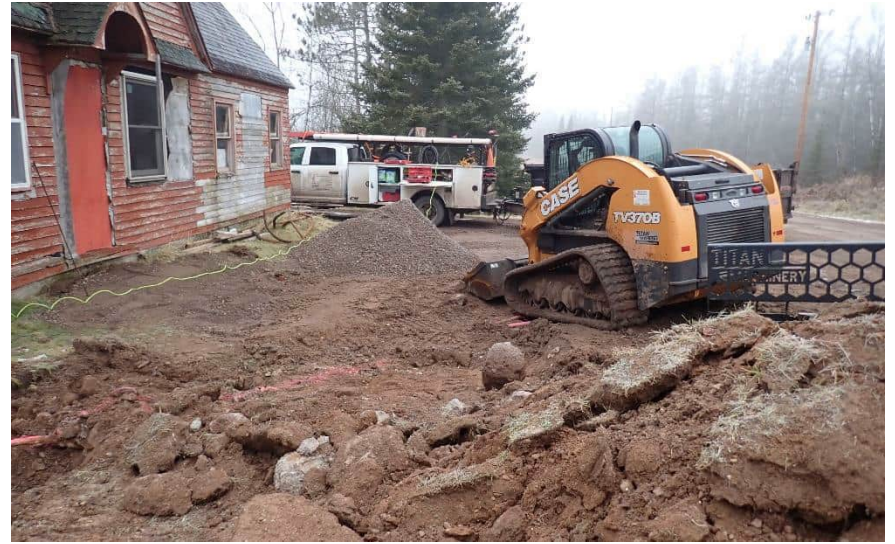
Area around excavation, facing west.
