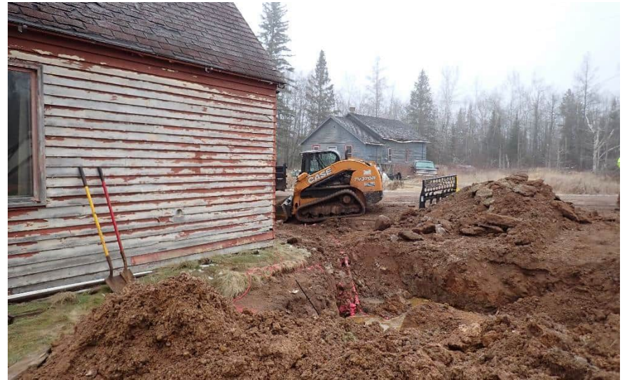
Excavation area, facing northwest.
