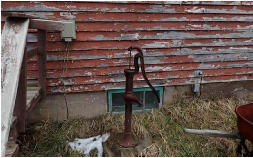
Well along western side of structure.
