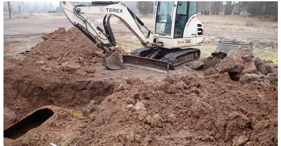
Area surrounding excavation, facing northeast.
