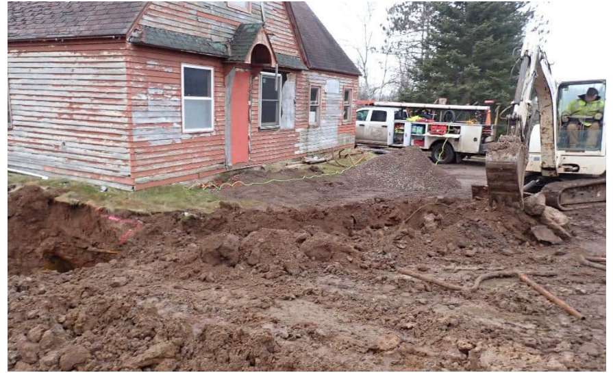
Trench to remove former dispenser piping, facing southwest.
