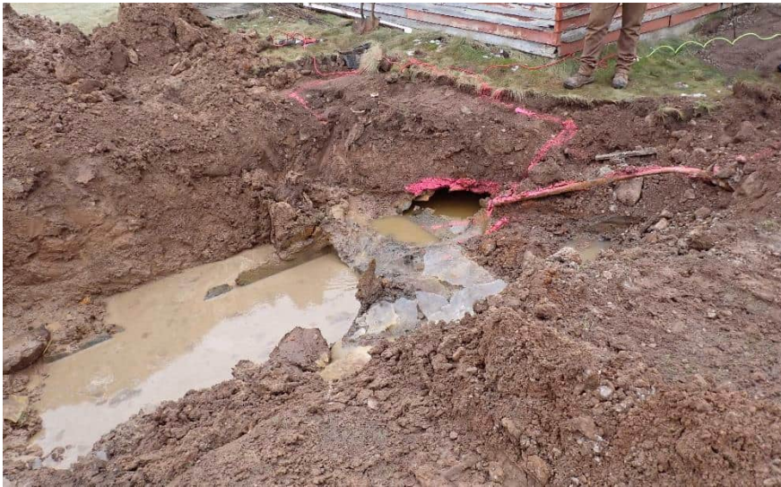
Excavation after 750-gallon tank was removed.
