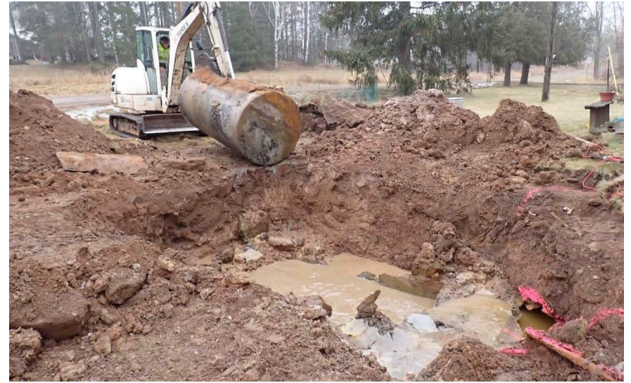
Removal of 750-gallon tank, facing southeast.
