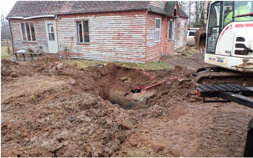
Excavation area before removing 550-gallon tank, facing southwest.
