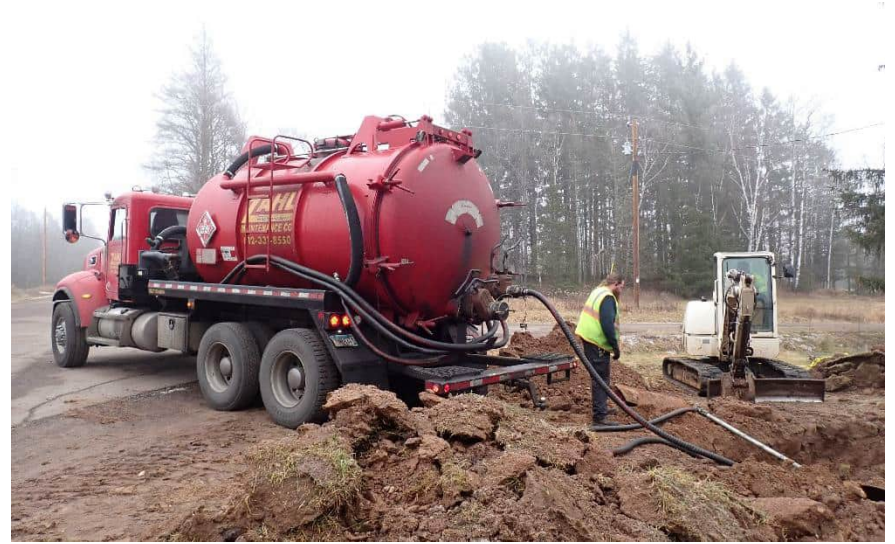
Vac truck removing liquid from excavation, facing east.
