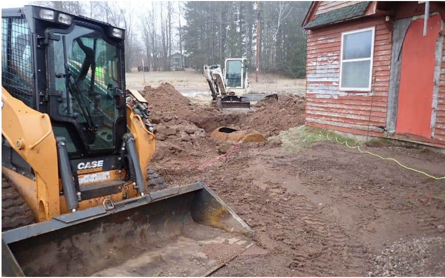
Front of structure and excavation area, facing east.
