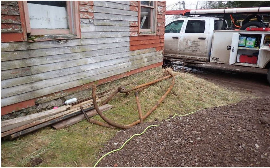
Removed piping from former dispensers.
