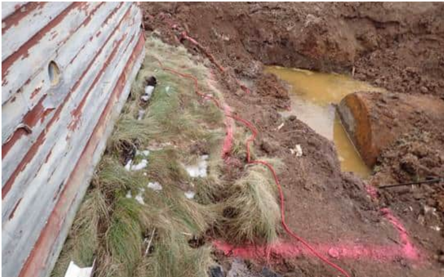
Northeast corner of structure and outline of 550-gallon tank.
