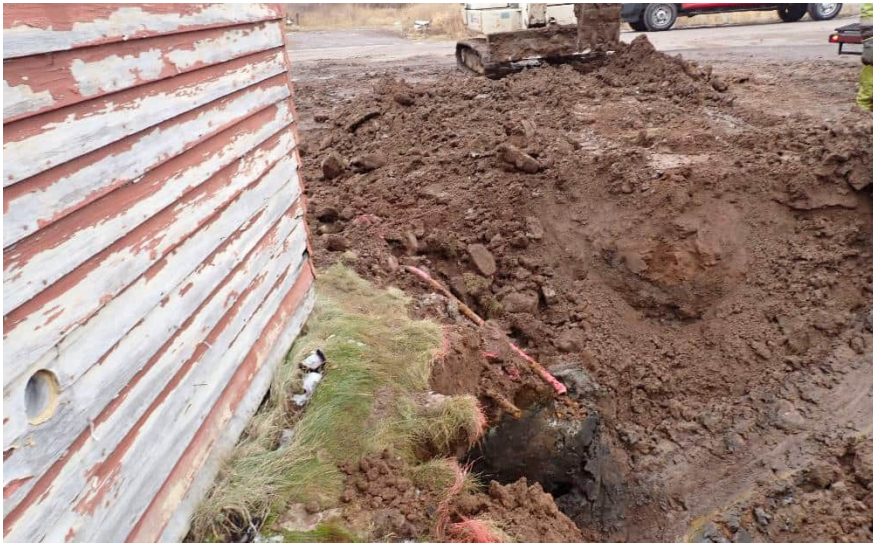
Northeast corner of structure and excavation area.
