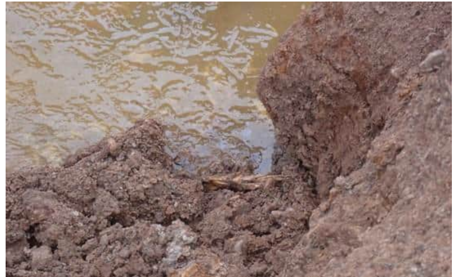
Slight sheen observed within excavation.
