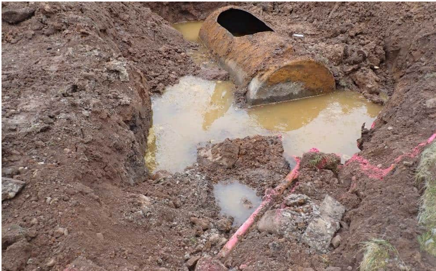
Excavation area and piping.
