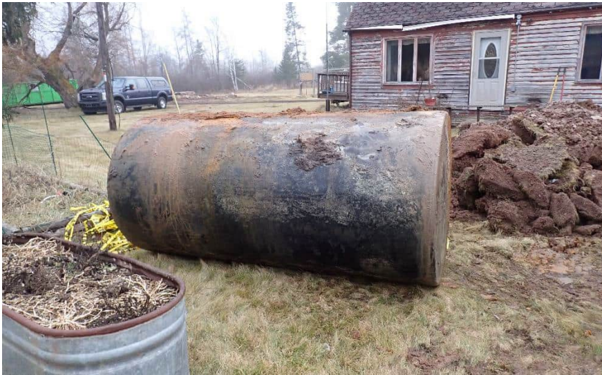
Removed 750-gallon tank, facing west.
