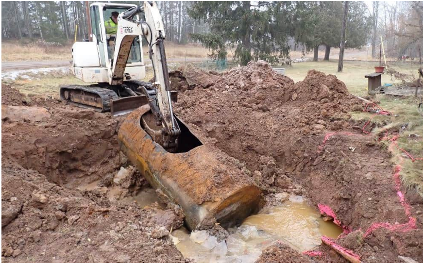
Removal of 750-gallon tank, facing southeast.
