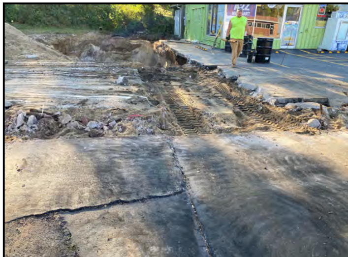
Piping run, view to south
