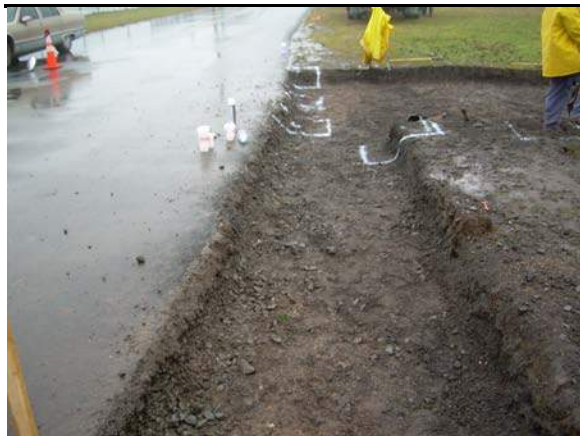
Picture 1: Sidewalk excavation and bollard layout
