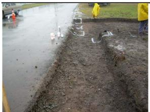
Picture 1: Sidewalk excavation and bollard layout
