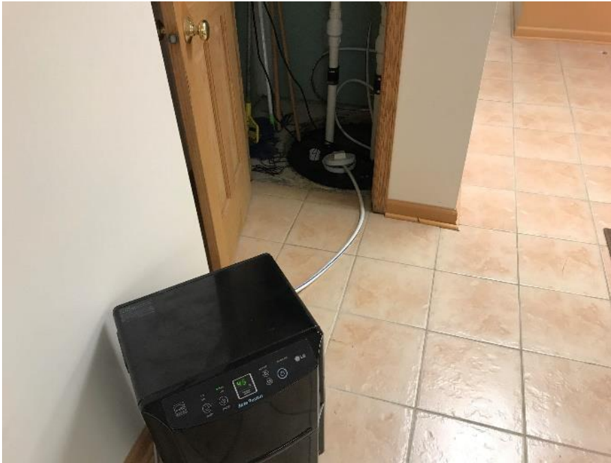
Photo 18: Sump 2 lid with open port for dehumidifier hose 08/06/2019
