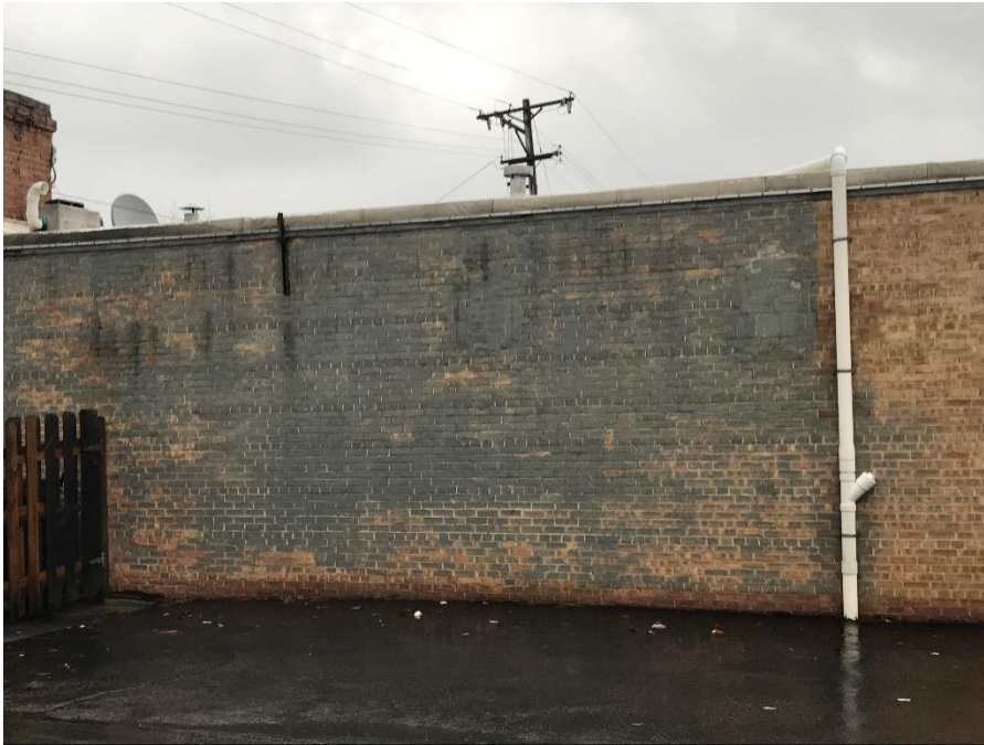
Photo 2: Sub-slab depressurization mitigation system vacuum lines on north side of Grace 1/07/2019
