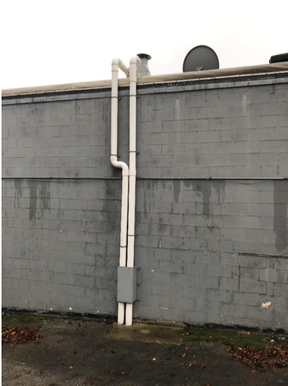
Photo 2: Sub-slab depressurization mitigation system vacuum lines on north side of Grace 1/07/2019
