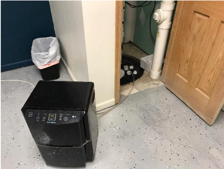
Photo 16: Sump 1 lid with open port for dehumidifier hose 08/06/2019
