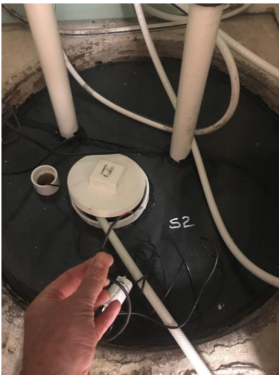
Photo 18: Sump 2 lid with open port for dehumidifier hose 08/06/2019
