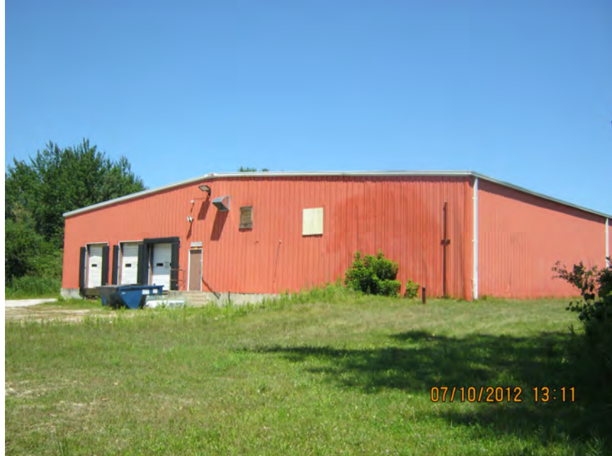
Photo 2: View of the eastern-most Lesperance subject property parcel building from the southwest. The potential UST vent pipe is visible on the southwest corner of the building.
