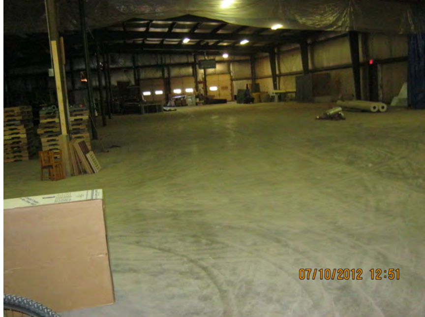
Photo 4: View of the warehouse area of the eastern-most building on the Lesperance parcel.
