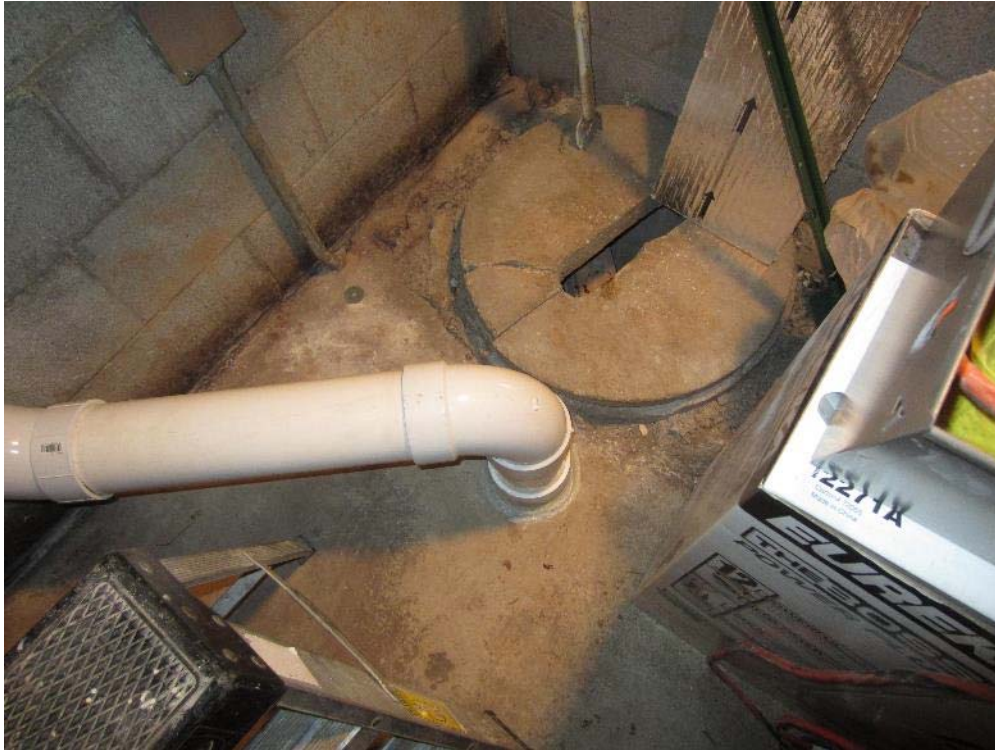
Photo 1: Northwest furnace room extraction point
