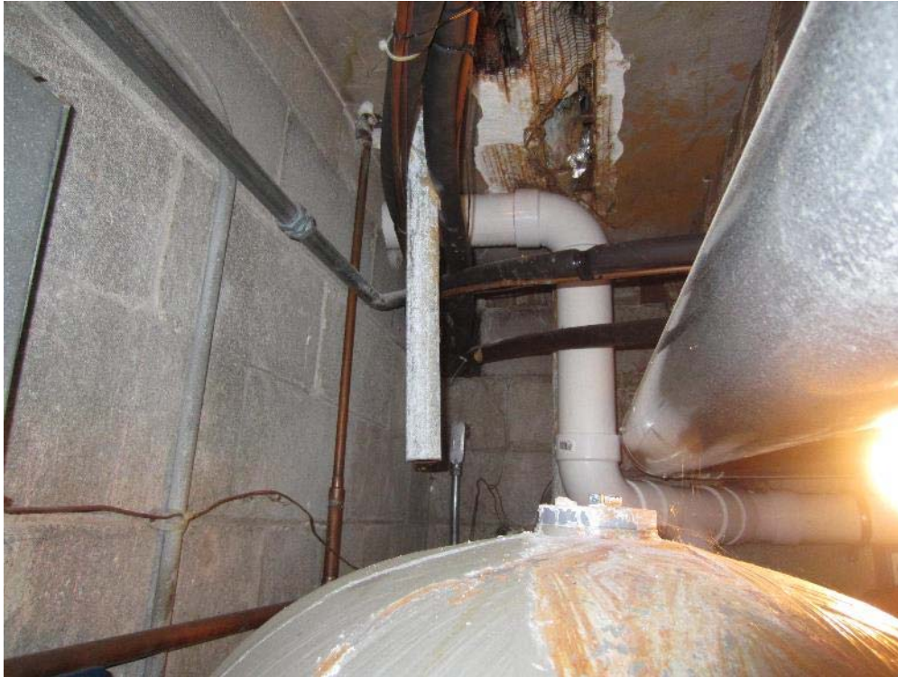
Photo 7: Southwest utility room wall penetration
