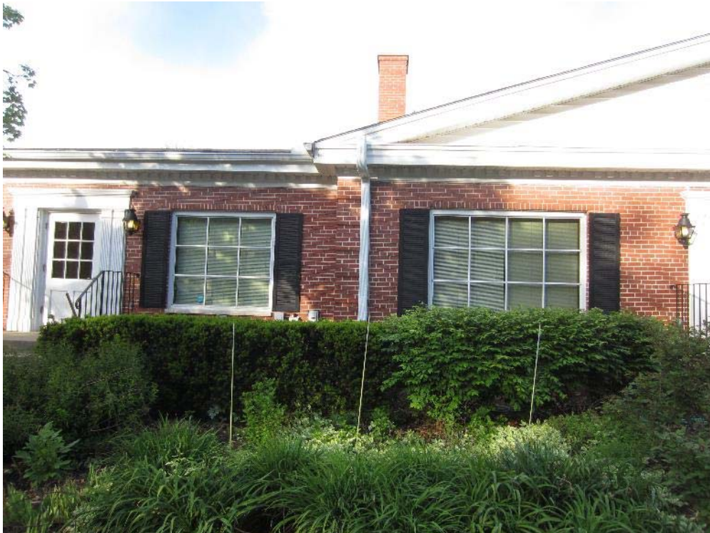
Photo 4: Northwest system exhaust
