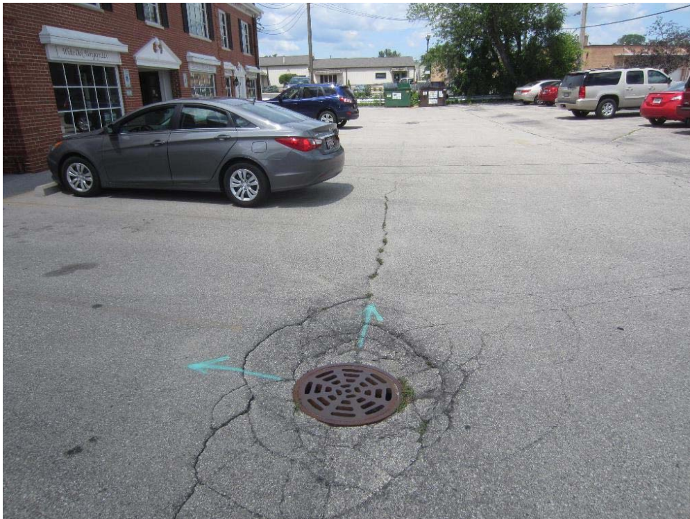
Photo 4: East parking lot facing north
