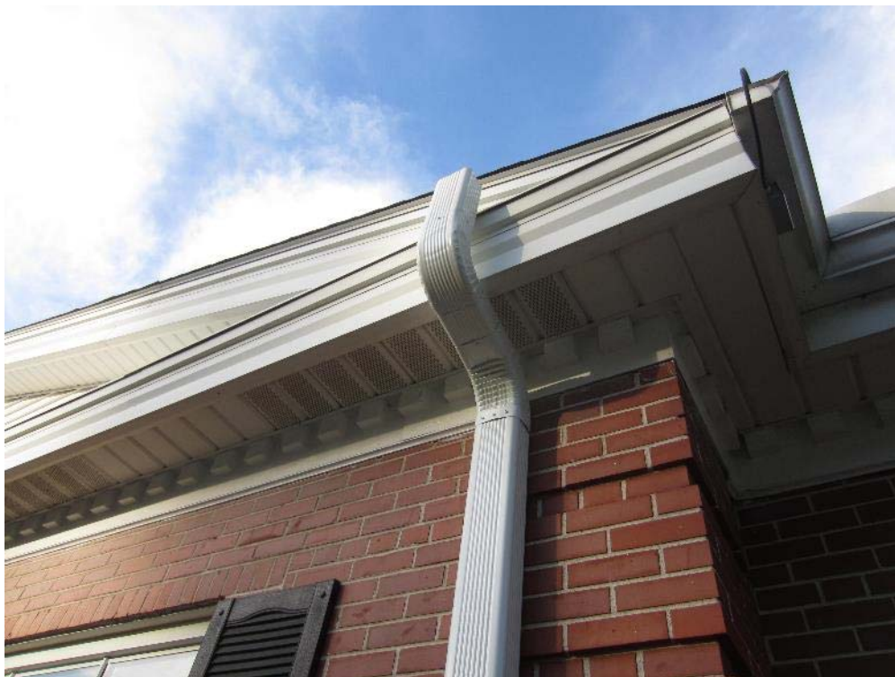
Photo 10: Southwest system exhaust location
