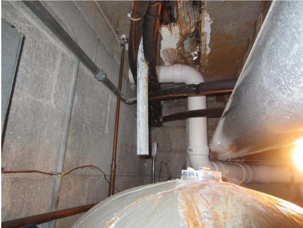
Photo 7: Southwest utility room wall penetration
