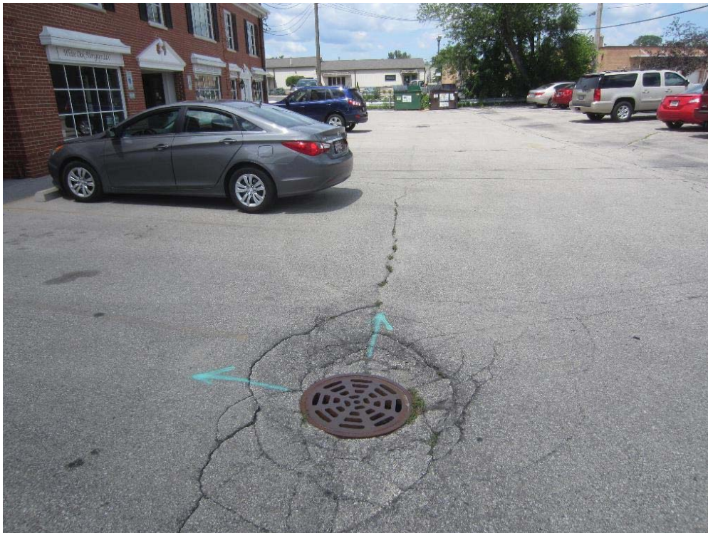
Photo 4: East parking lot facing north
