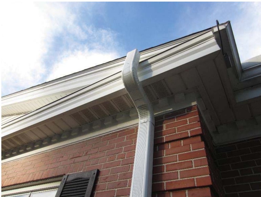
Photo 10: Southwest system exhaust location
