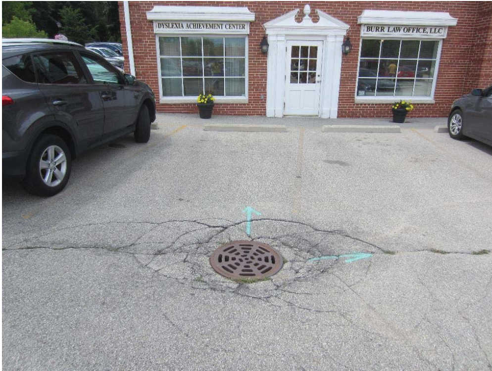
Photo 3: East parking lot facing west
