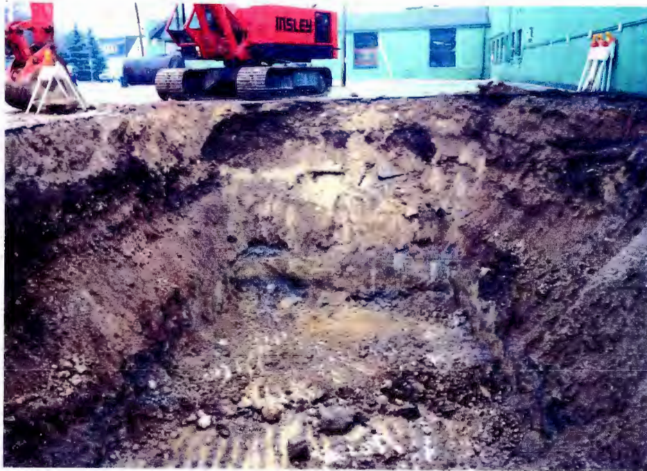
Excavation looking east -- contaminated zone is above bedrock.
