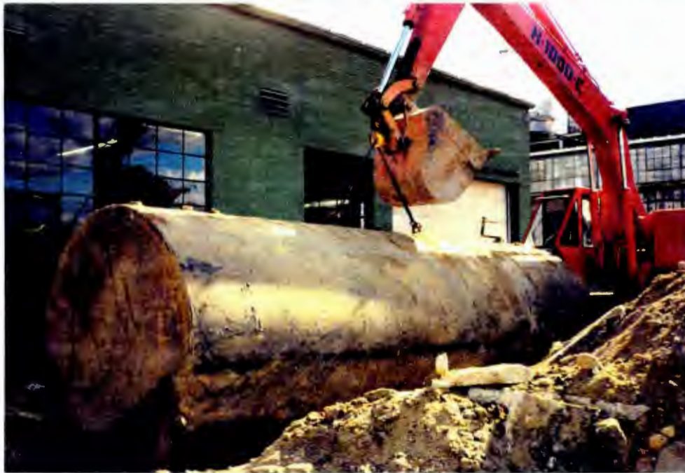
Removal of the 12,000 gallon diesel tank.
