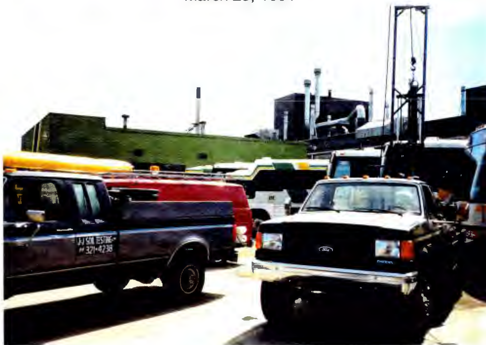
Drilling SB-21 March 28, 1991
