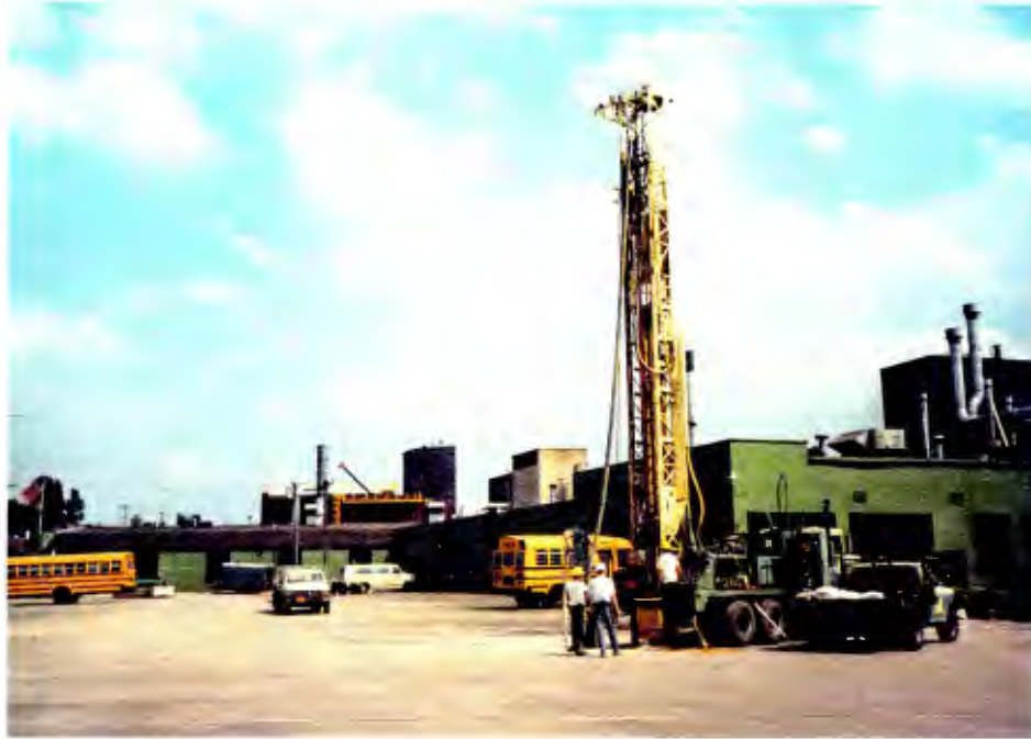
Drilling SB-39/MW-6 May 30, 1991
