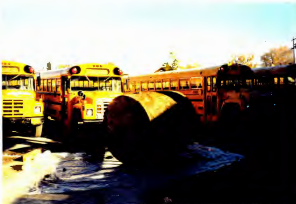
1000 gallon waste oil tank after removal.
