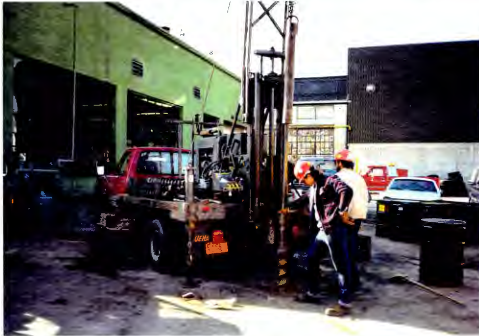
Drilling SB-15 March 25, 1991
