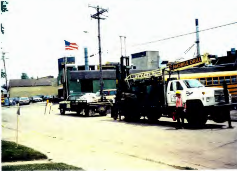
Drilling SB-35 in street. May 29, 1991
