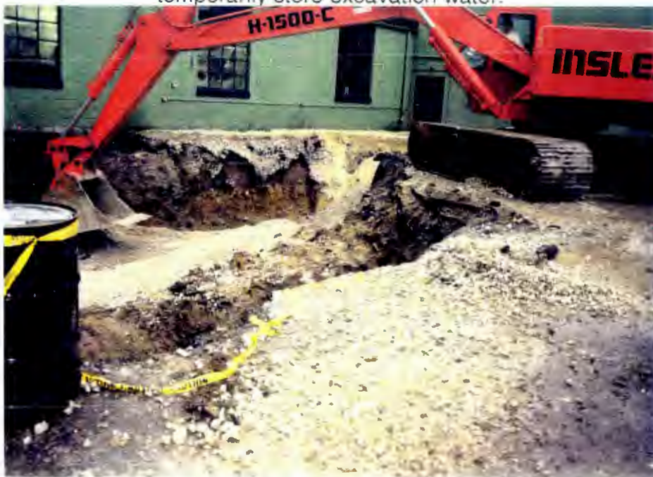
Spreading gravel backfill in south end of excavation.
