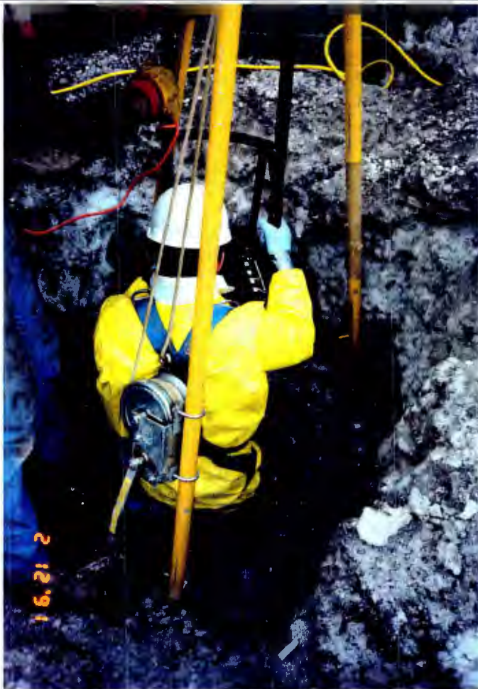
Entering 6000 gallon diesel tank to obtain soil sample. February 12, 1991
