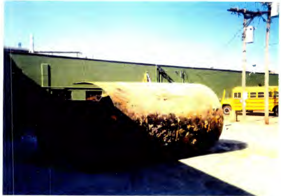
The 6000 gallon diesel tank after removal from south end of excavation. June 19, 1991
