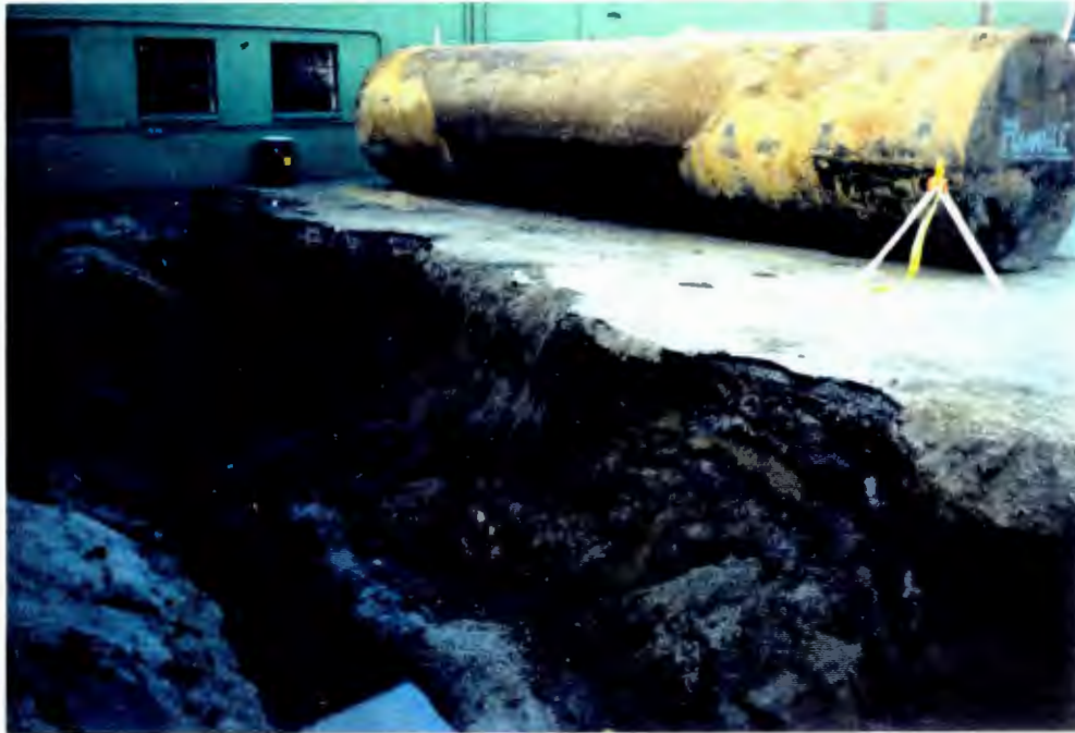
15,000 gallon gasoline tank after removal. 6000 gallon diesel tank still in ground..
