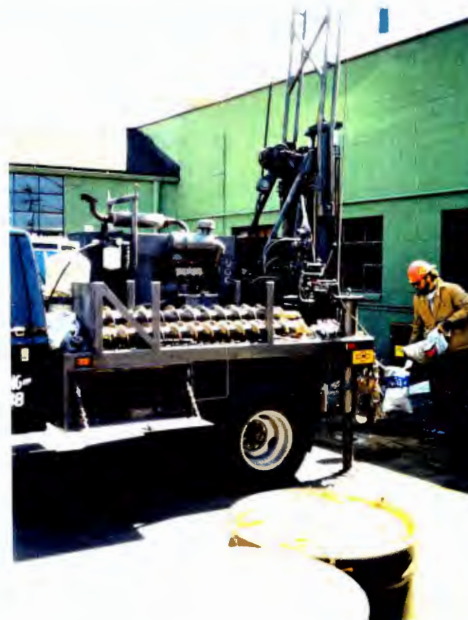
Drilling SB-31/MW-4 April 1, 1991
