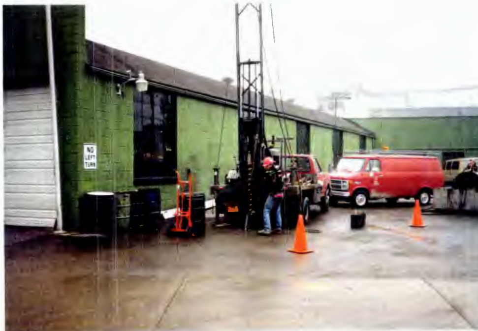
Drilling SB-13 March 22, 1991
