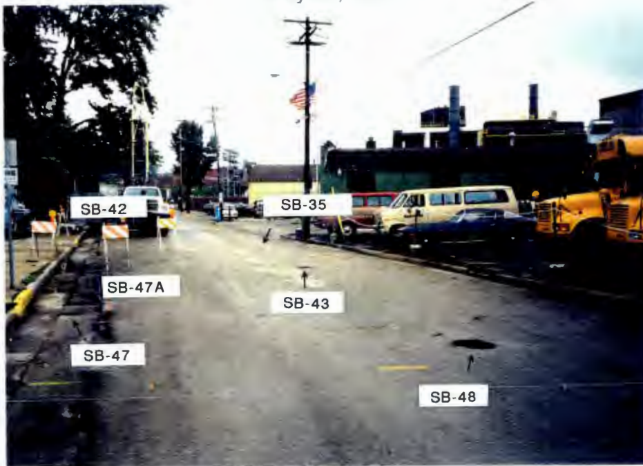
Drilling SB-49 in street. July 12, 1991
