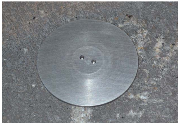
Figure 4. Secure Cover Installed
