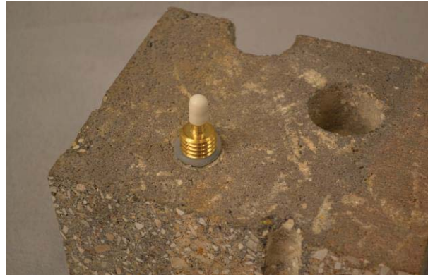
Figure 3. Installed VAPOR PIN®
