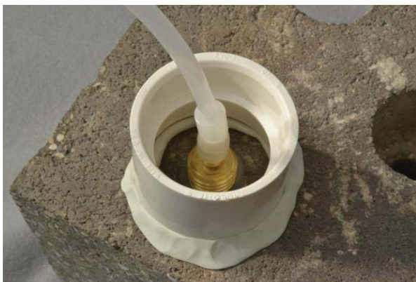
Figure 6. Water dam used for leak detection
