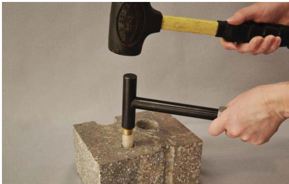
Figure 2. Installing the VAPOR PIN®
