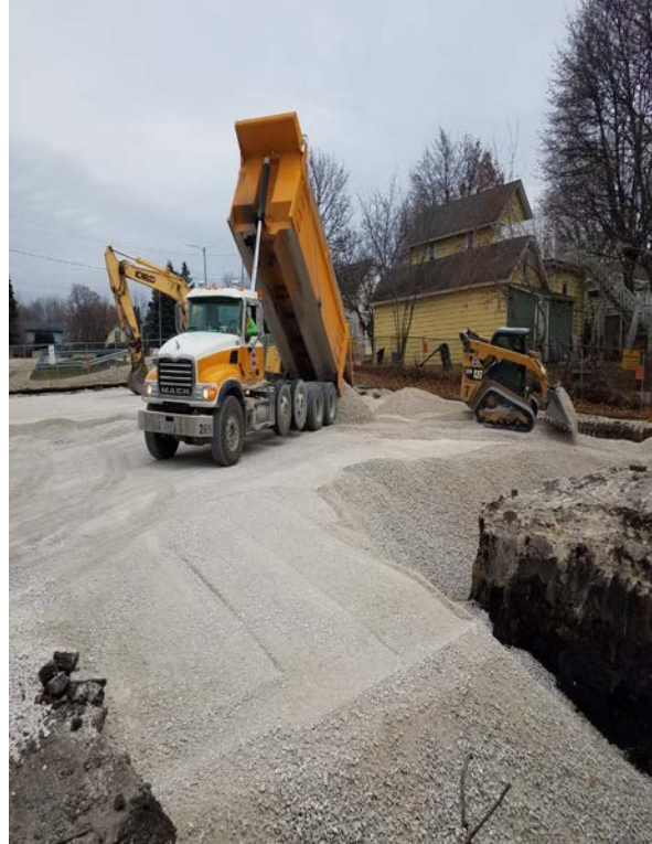
14. Ongoing backfill operation. Looking SE.
