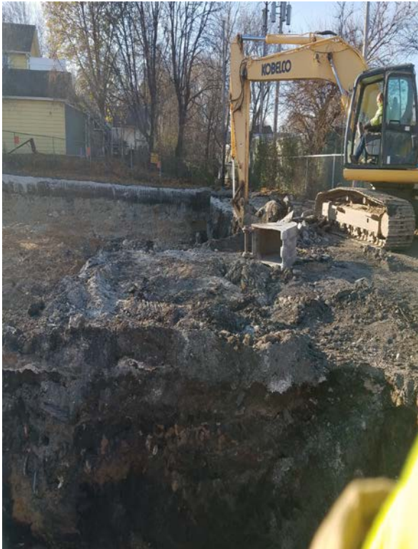
9. Excavating west side. Looking S.
