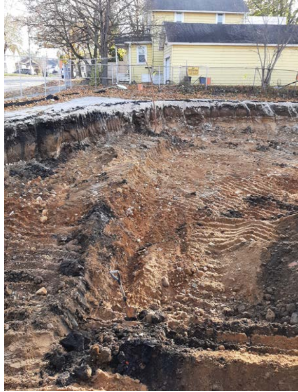
6. Ongoing excavation. Looking S.
