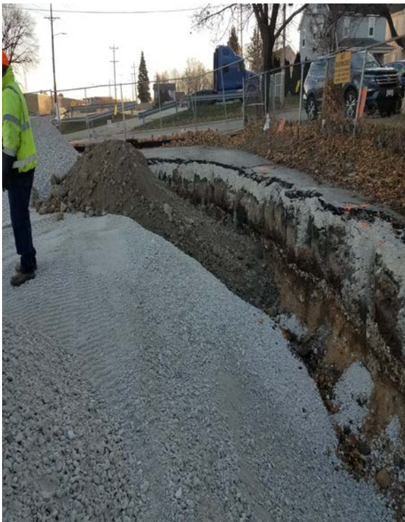
15. Placement of clayey backfill along southern excavation border. Looking E.
