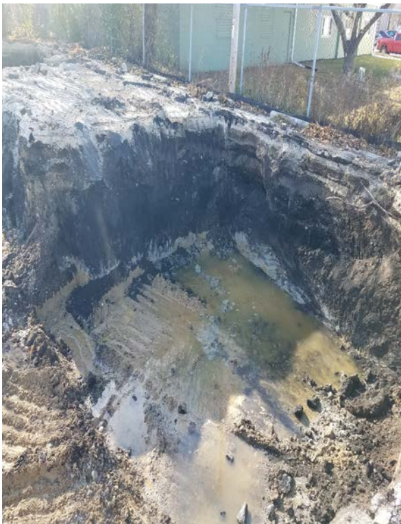
11. Grid excavated to groundwater. Looking SW.
