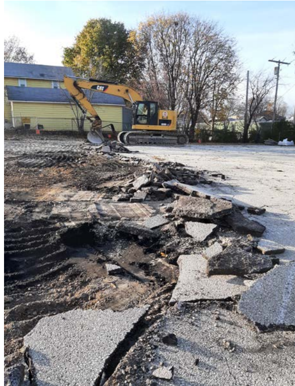
2. Asphalt removal. Looking S.
