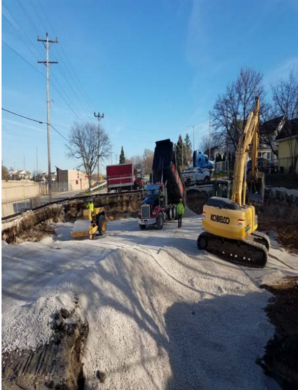
13. Backfilling operations. Looking E.
