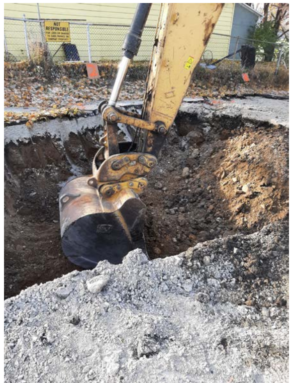
4. Start of excavation activities. Looking S.
