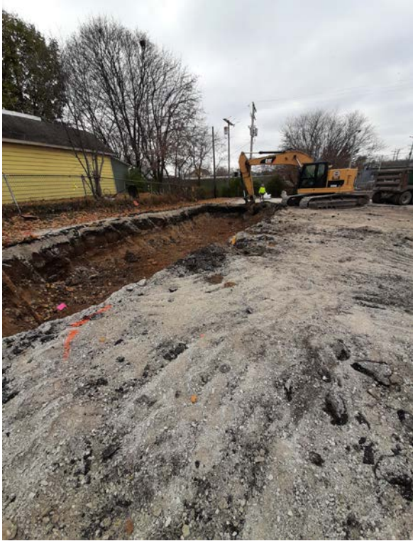
5. Excavating along south edge. Looking W.
