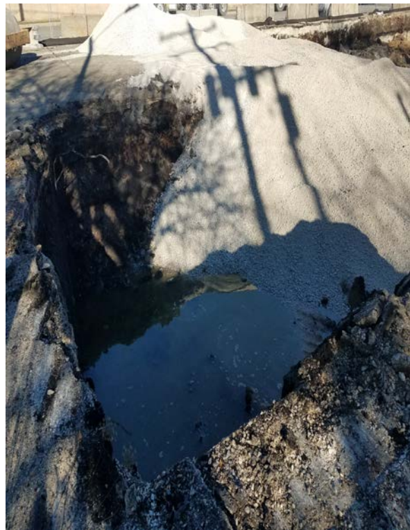
12. Start of fill import for backfilling. Looking N.
