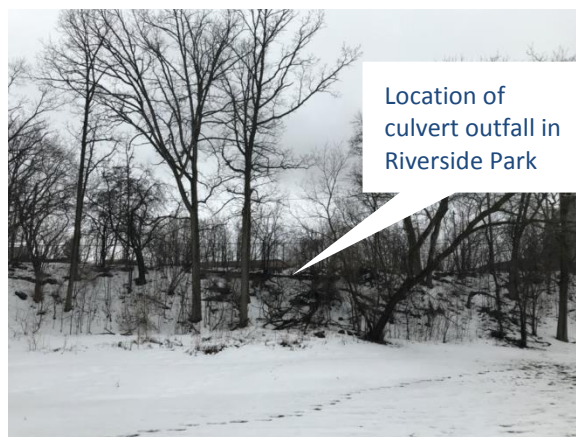
Figure 3. Culvert location at Riverside Park
