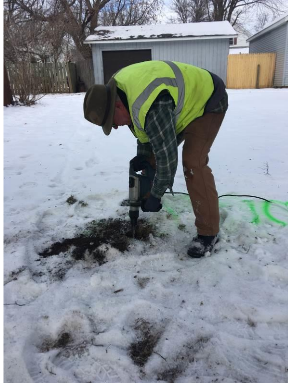
Photo No. 5 B-103 using hammer drill
