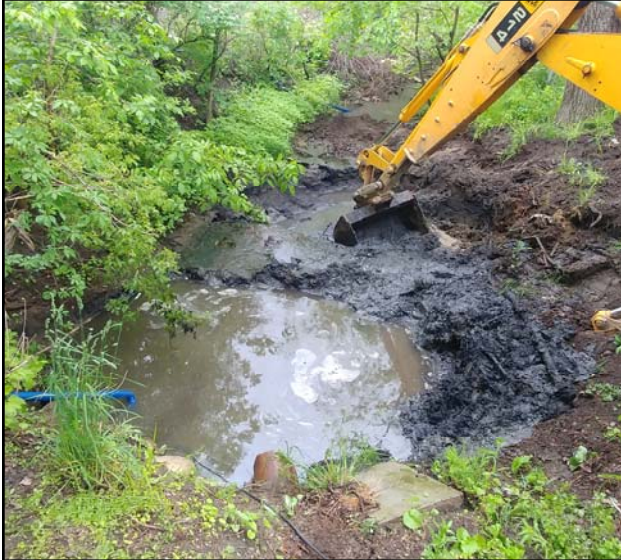
Photograph 1 - Drainage swale during limited soil removal.
