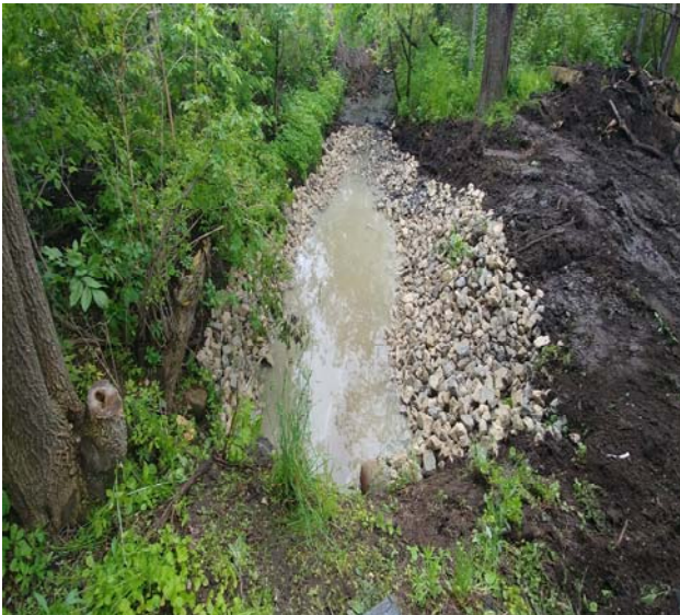
Photograph 3 - Drainage swale after limited soil removal and placement of stone.
