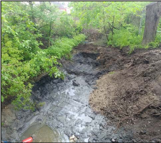
Photograph 2 - Drainage swale after soil was removed
