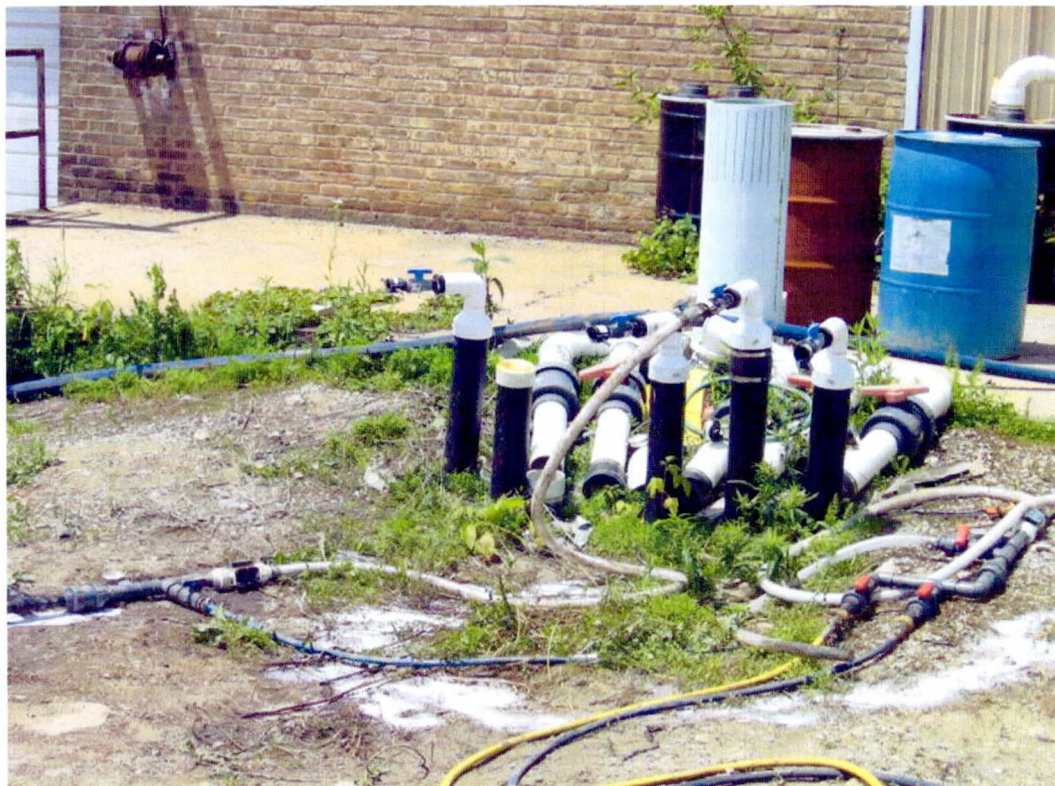
Photo 8 – Injecting EOS into SVE lateral piping.
