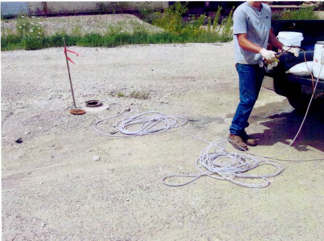
Photo 12 – Injecting BAC-9 at TW-02.
