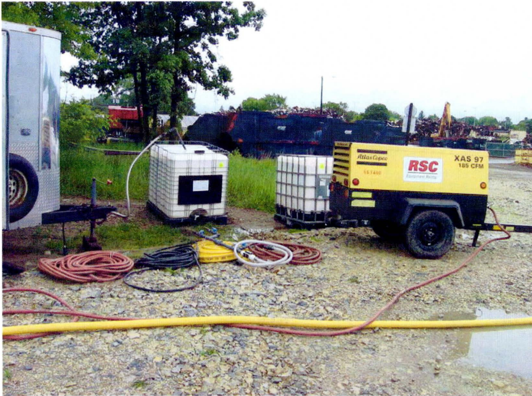
Photo 10 - EOS totes and equipment used for injection at L1 treatment area.
