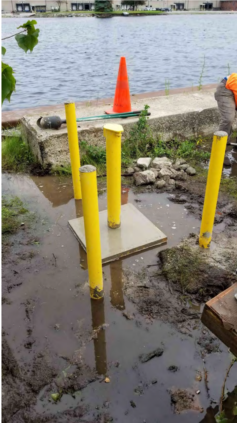
Photograph 2: MW122S completed well pad and bollard installation
