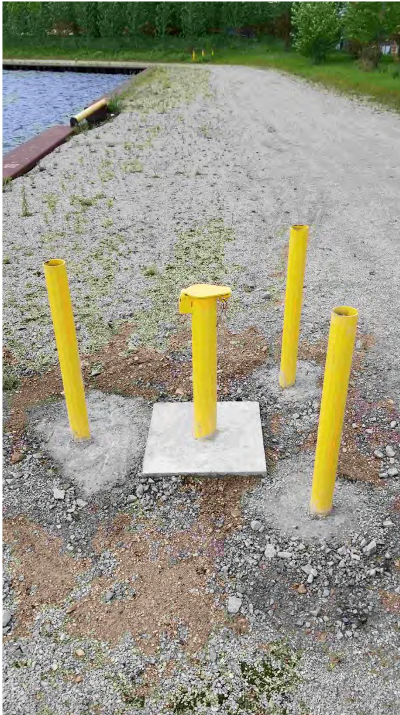
Photograph 3: MW123S completed well pad and bollard installation
