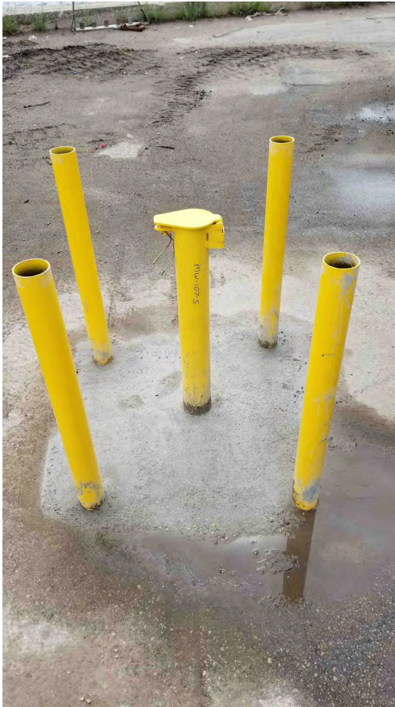
Photograph 5: MW107S completed well pad and bollard installation
