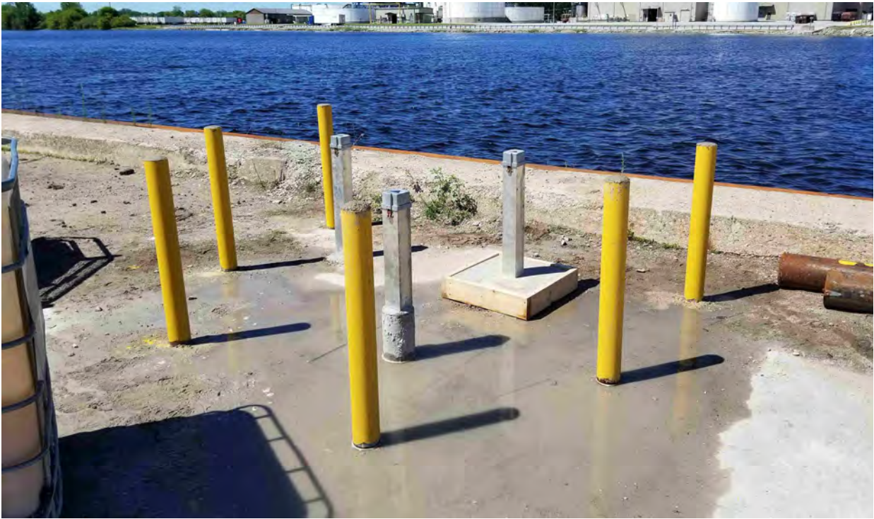
Photograph 6: MW118D-R well installation and MW118S and MW118M well repairs
