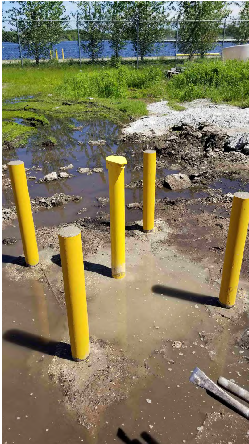
Photograph 7: MW068S well repair
