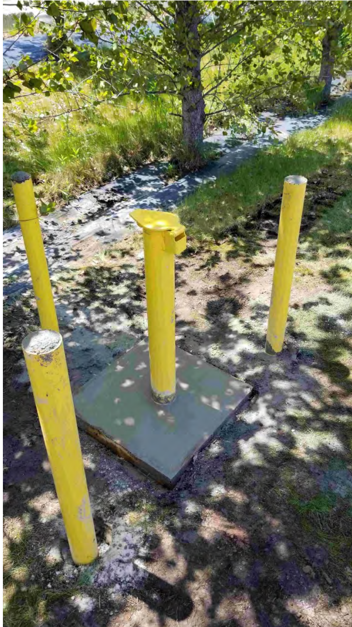
Photograph 1: MW121S completed well pad and bollard installation
