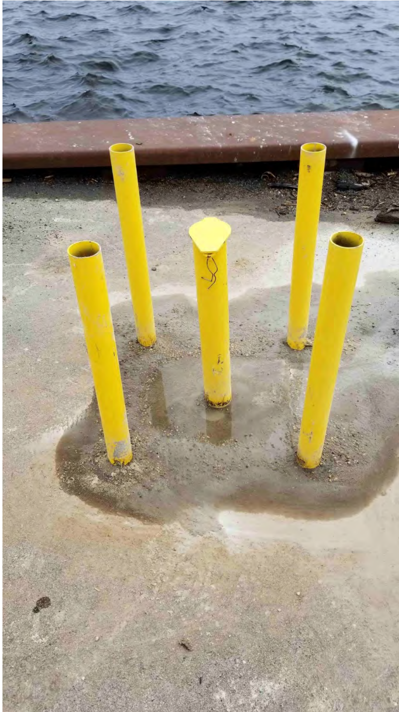
Photograph 4: MW124S completed well pad and bollard installation
