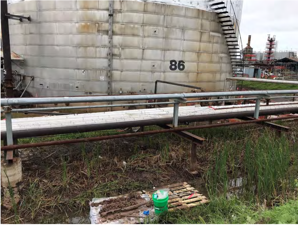
Photo 5: HA-2; boring location adjacent to standing water; facing north
